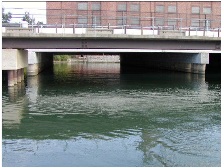
General Elevation View
