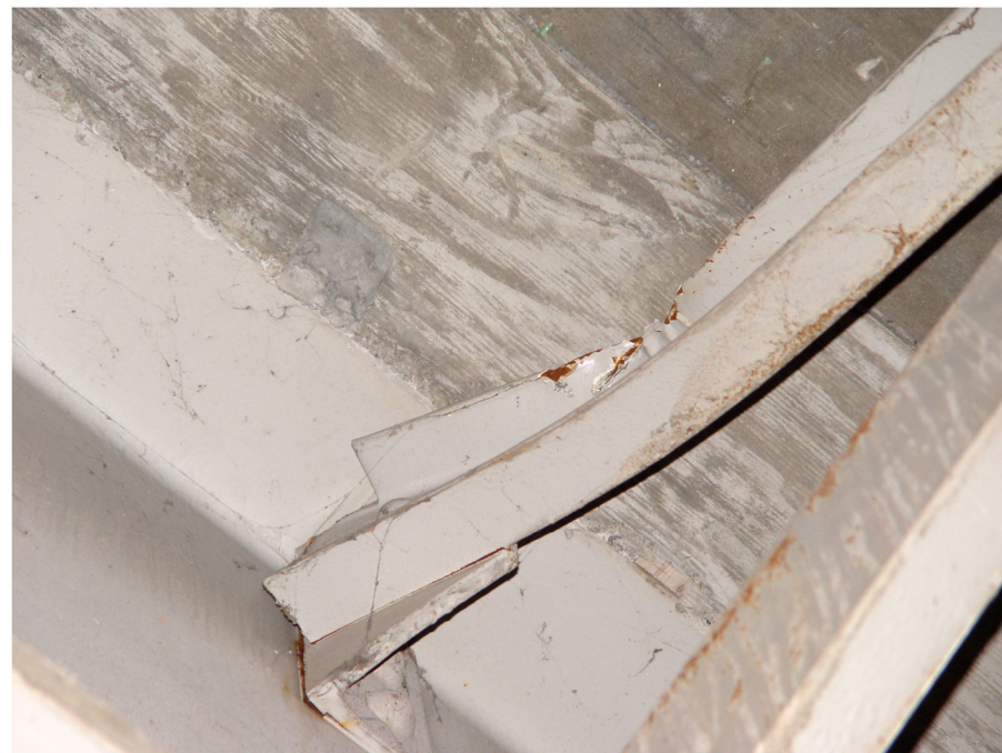
1808745 10_5_05 P4 bent crossframe channel.jpg
