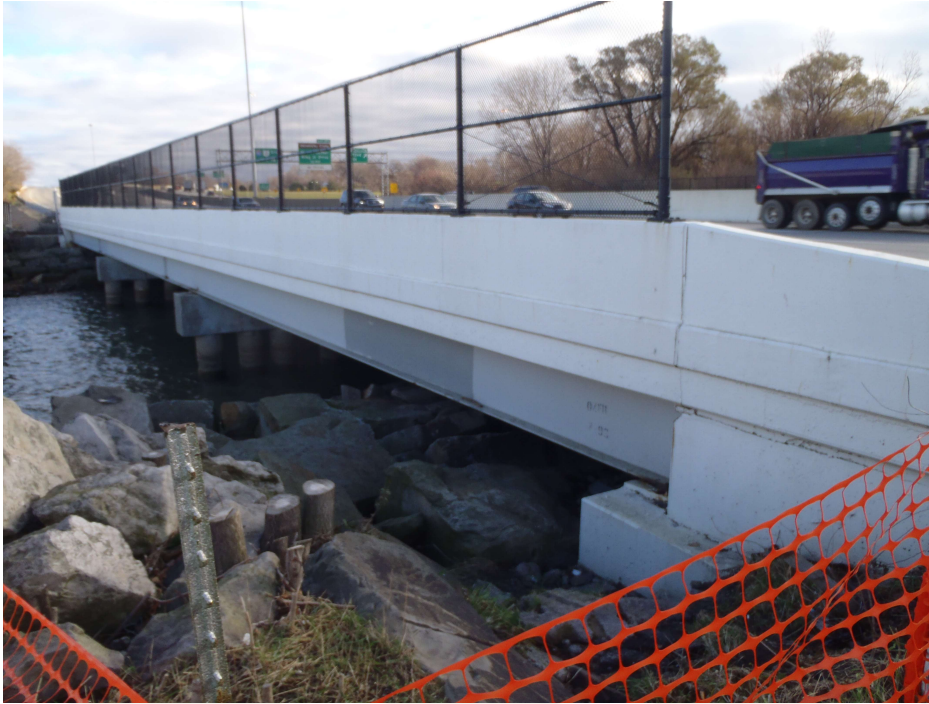
Photo 1 - Downstream (North) Fascia Looking South
