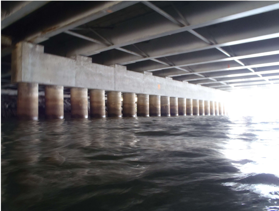
Photo 2 - Typical Bent Configuration, Bent 1
