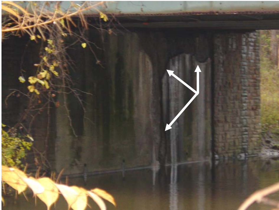
Photo 3 - Facing West. View of Start (west) Abutment. Note large spalled area below drain.
