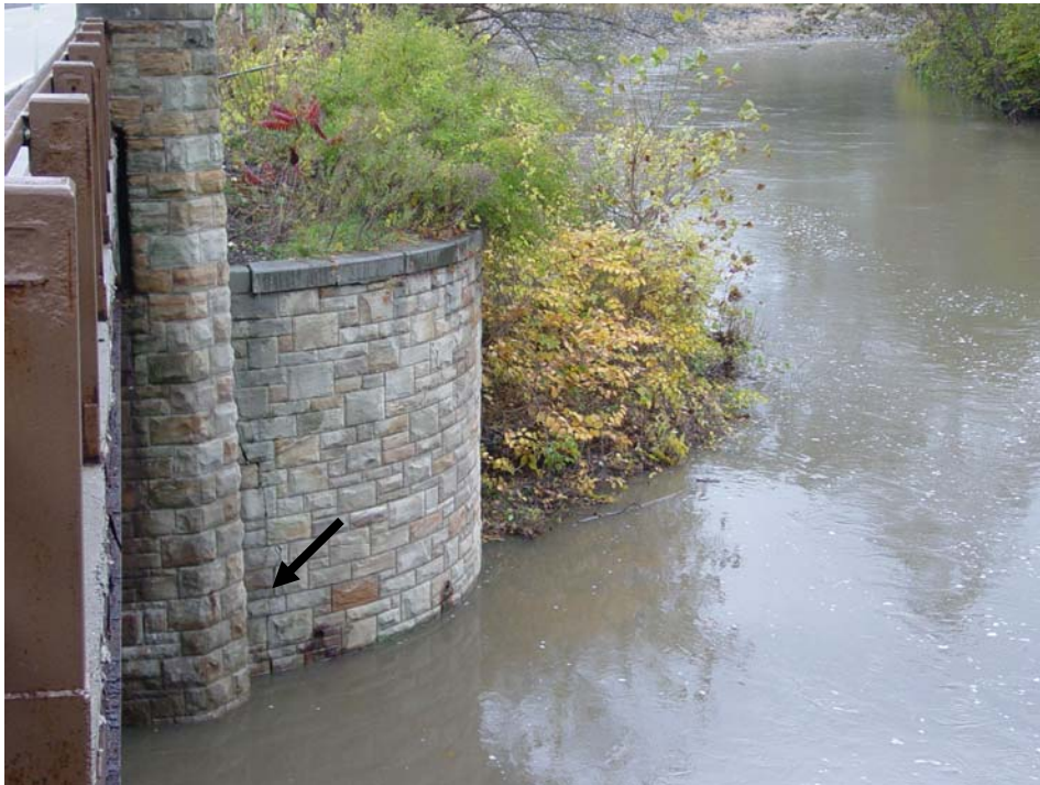
Photo 6 - Facing East and looking upstream. View of Finish Right (southeast)Wingwall. Note full height crack (3/8" wide).
