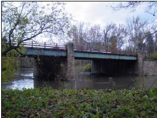
General Elevation View
