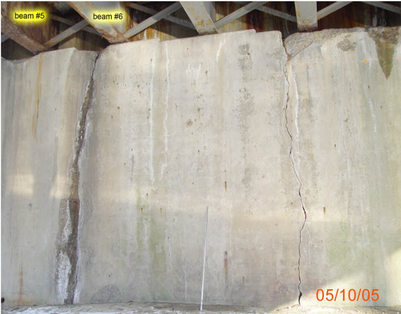
P10: FINISH ABUTMENT CRACKS.
