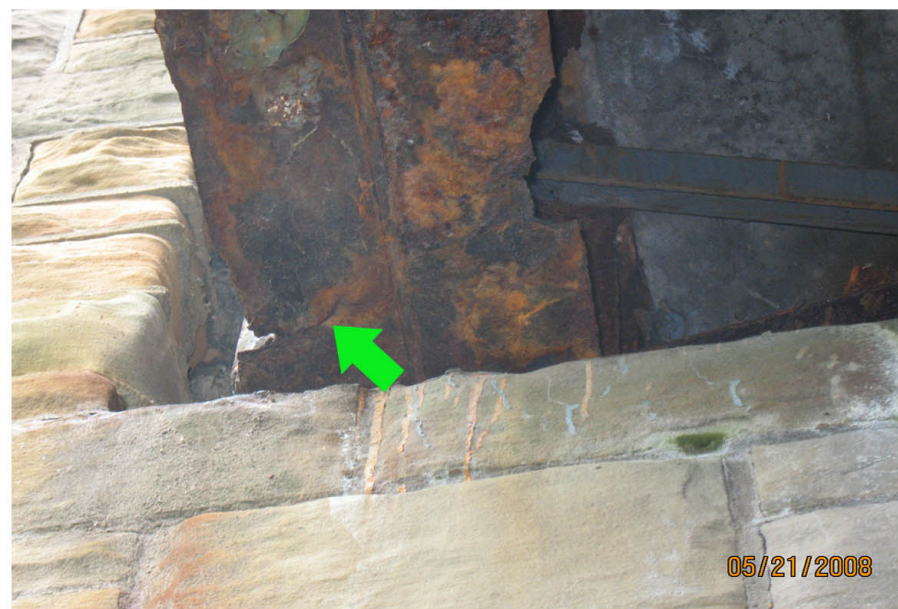
P6: ARROW POINTS TO CRACKED LOWER FLANGE OF RIGHT FASCIA AT THE START ABUT. NOTE SECTION LOSS TO FLANGE.
