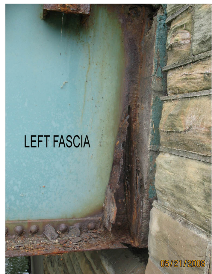
P7: RUSTED AWAY STIFFENER. RUST THRU HOLE TO LOWER FLANGE. THIS IS THE FINISH SIDE OF THE PIER.
