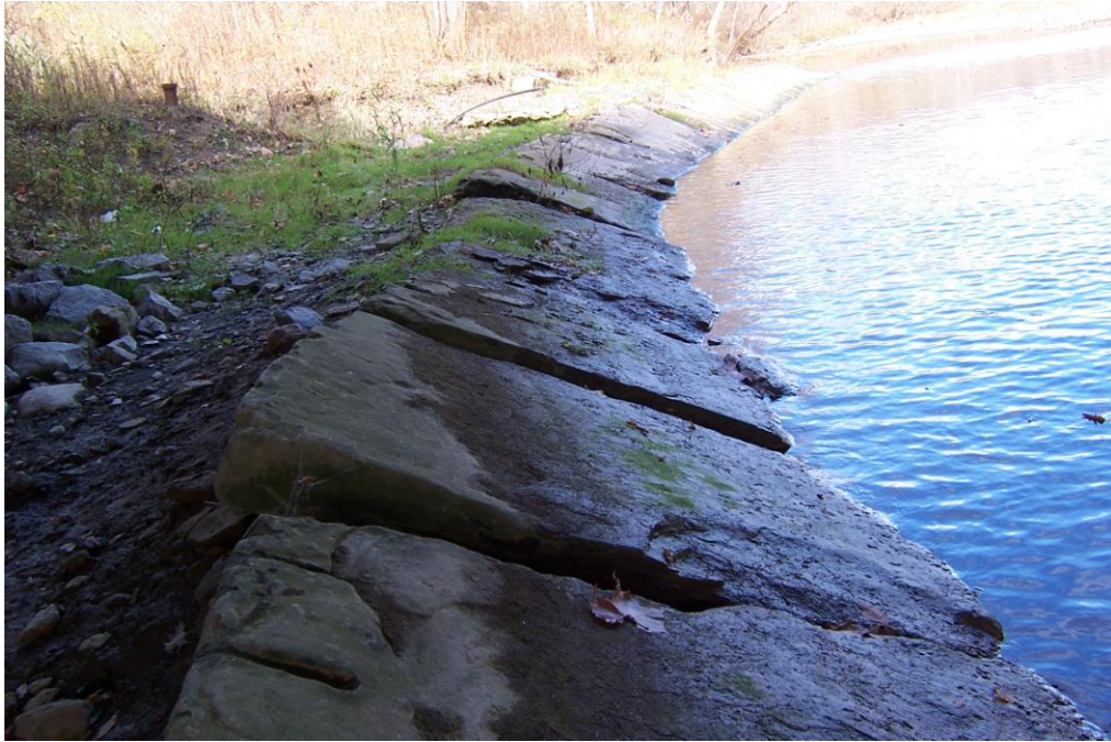
Photo 9 - Facing North. Large stones along the West Embankment for Scour Protection.
