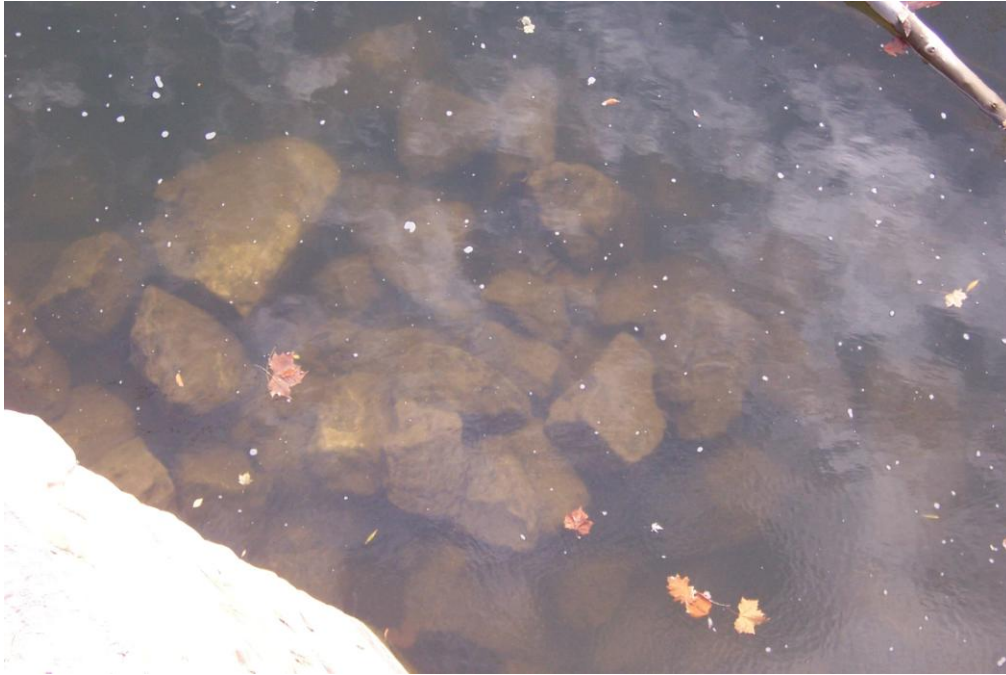
Photo 11 - Facing Downward. Riprap along the Pier (south end shown).
