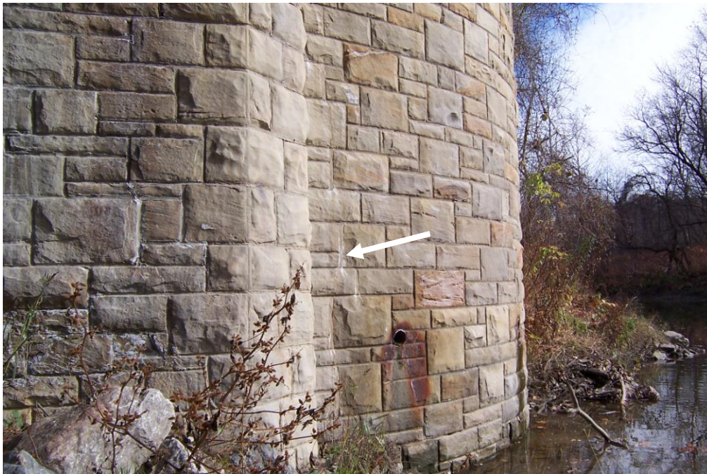
Photo 12 - Facing Southeast. Repaired Crack in the Southeast Wingwall.
