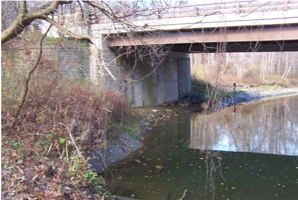
Photo 7 - Facing Northwest. West Abutment and missing shore protection.
