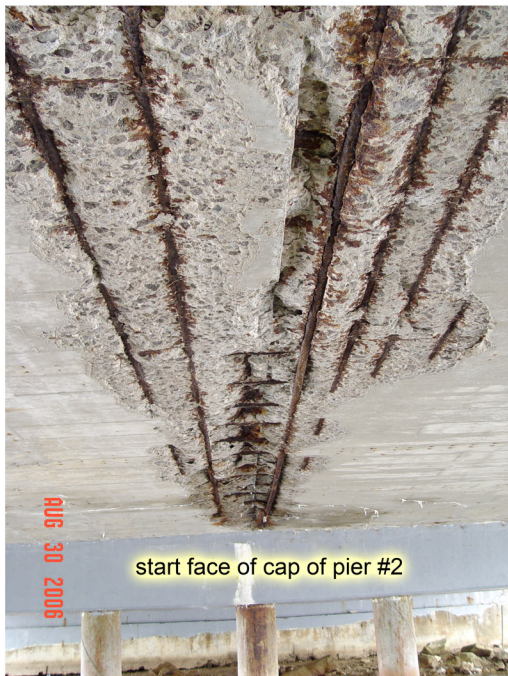
P3 360 degree exposure of slab rebars in span #2.psd
