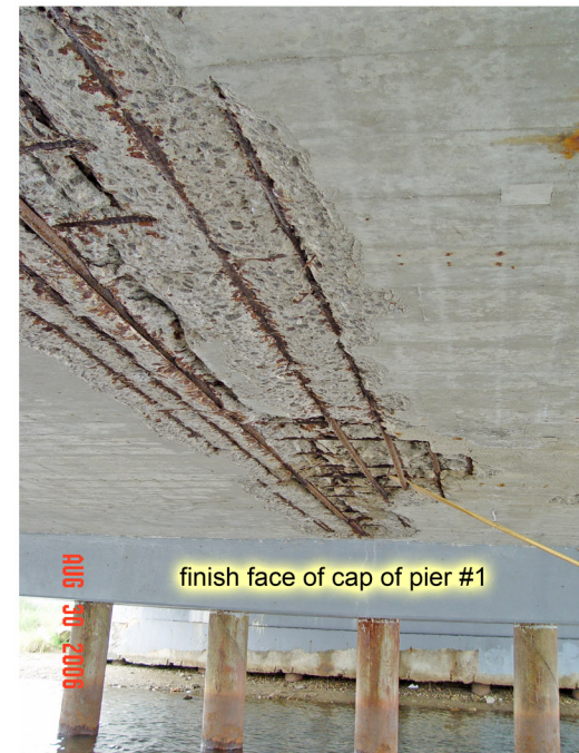
P4 360 degree exposure of slab rebars in span #2.psd
