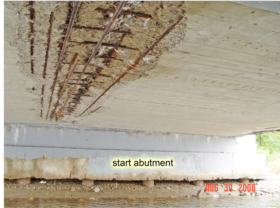
P2 360 degree exposure of slab rebars in span #1.psd
