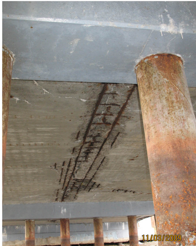
P2: SPAN #2 (MID) UNDER CENTERLINE.
