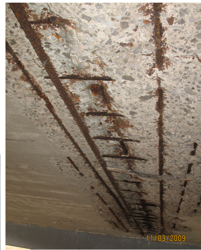
P3: SPAN #3 UNDER CENTERLINE.
