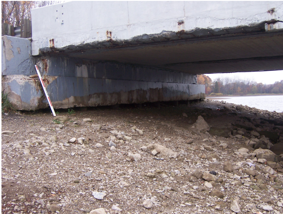
Photo 5 – Facing West. South Abutment with full width Undermining and Exposed Piles.
