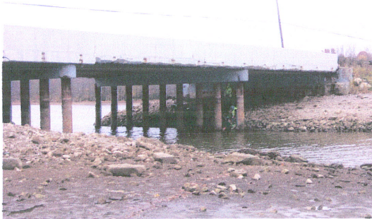
East Elevation View
