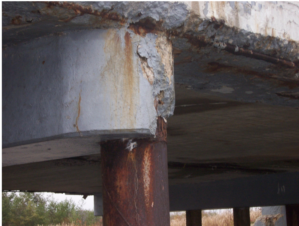
Photo 8 – Facing Southeast. West end of Pier 2 (North Pier) pile cap with Corner Spall.
