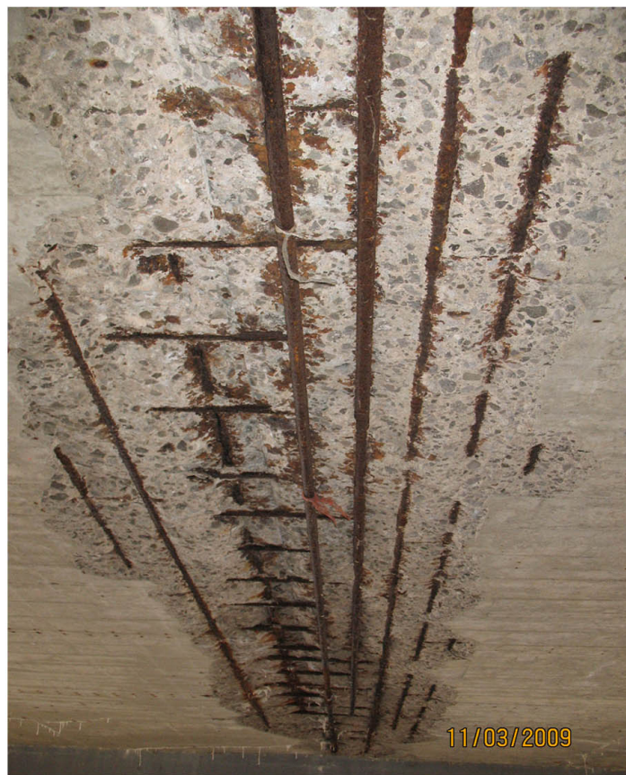
P1: SPAN #1 UNDER CENTERLINE OF BRIDGE.
