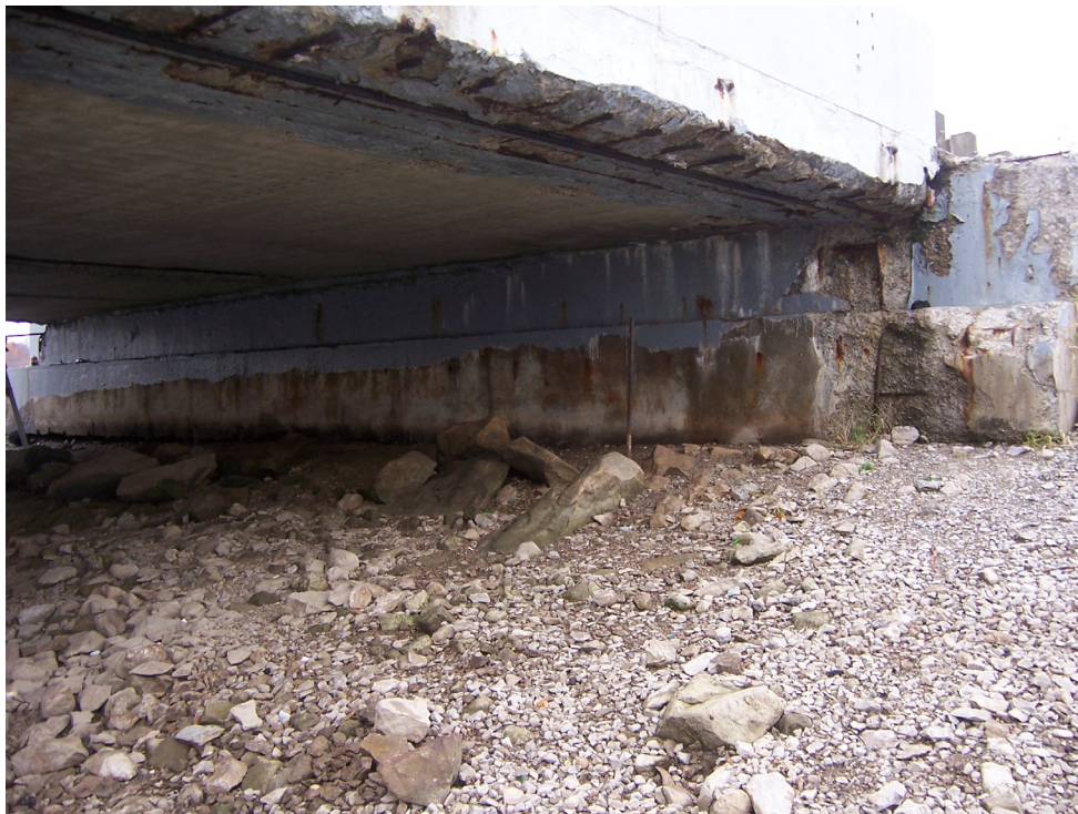
Photo 6 – Facing Northwest. North Abutment with West Corner Undermining.
