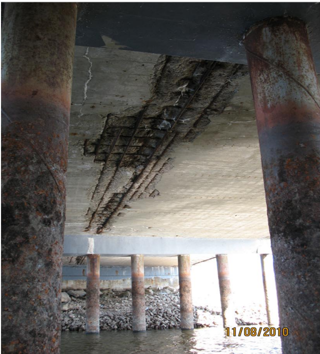
P3: LOOKING NORTH AT MID-SPAN.
