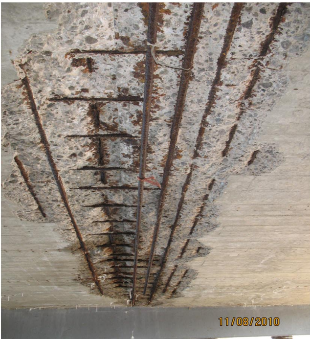
P1: LOOKING NORTH IN SPAN #1 (SOUTH SPAN)
