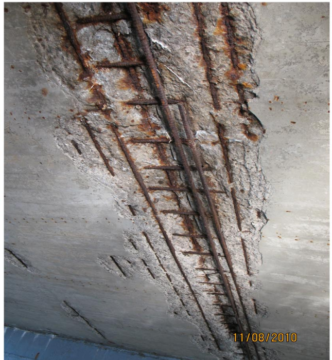
P4: LOOKING NORTH IN SPAN #3.
