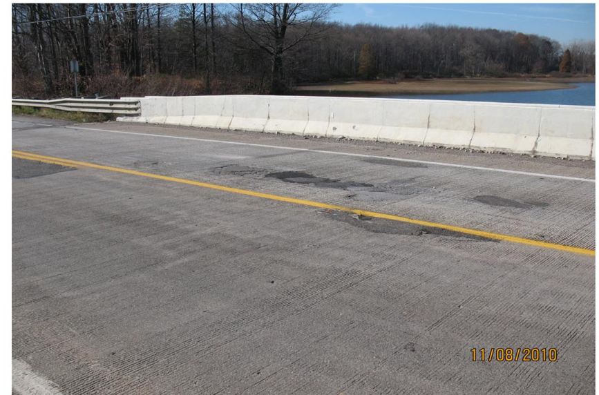
P8: ASPHALT PATCHES AND BREAKING UP AREAS OVER SPAN #1 AND PIER #1.
