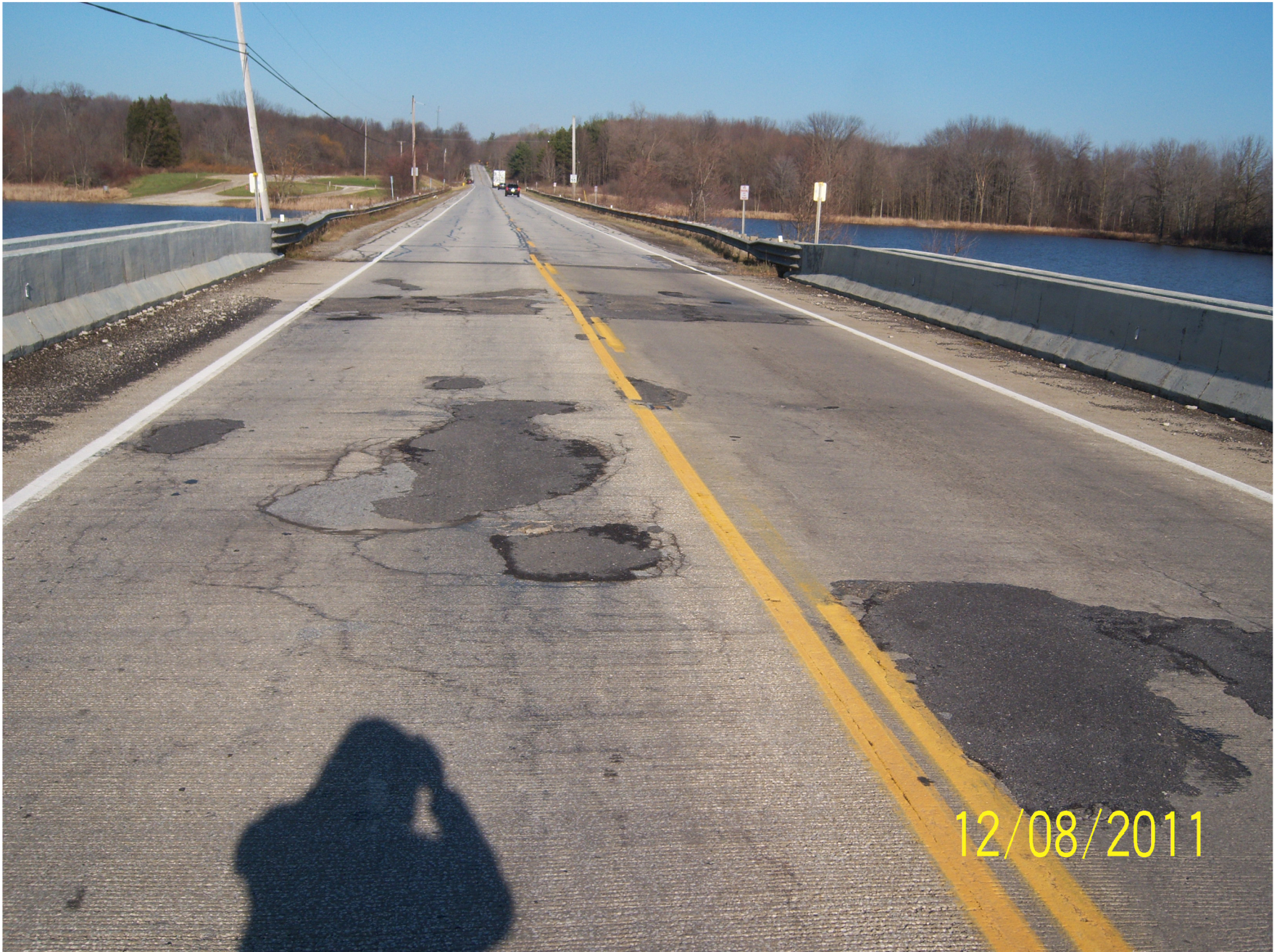
P6: Wearing surface viewed facing north from south end of deck.
