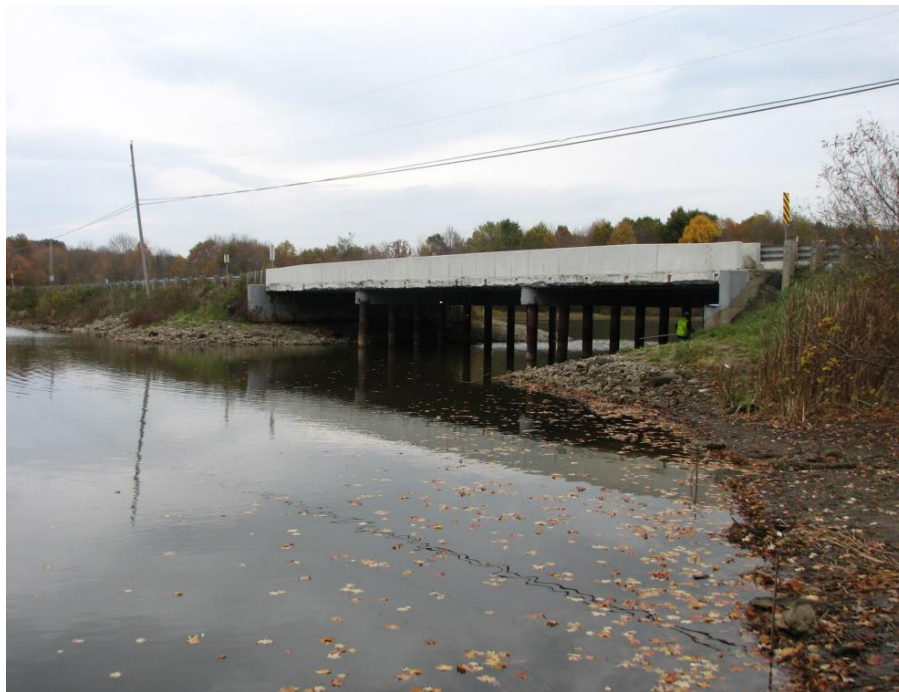
(West Elevation of Structure)
