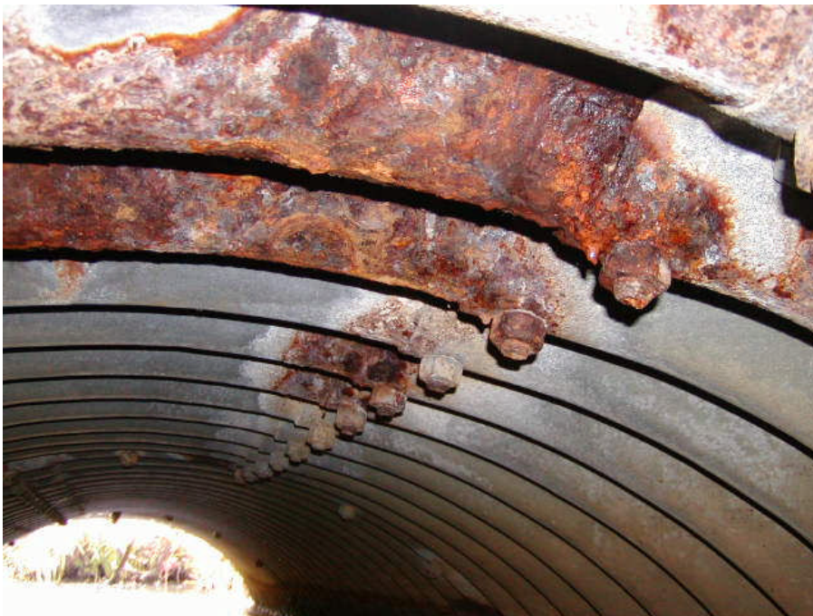
Photo 6. Typical surface corrosion on roof of culvert.
