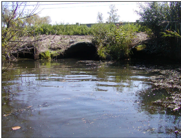
General Elevation View
