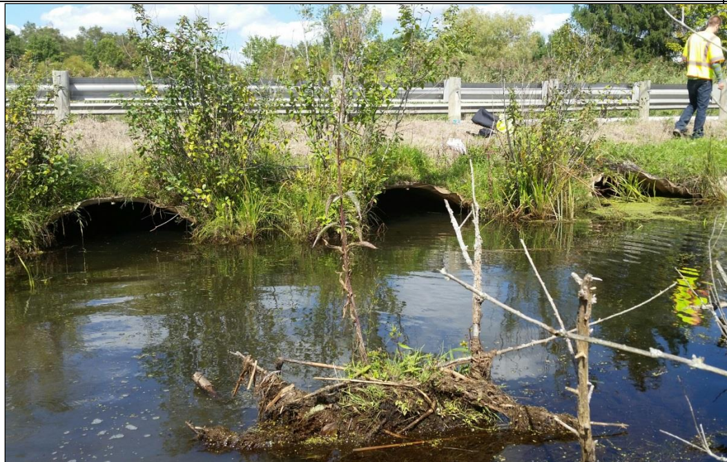
Photograph 2 Overall View of the South Elevation. Looking North.
