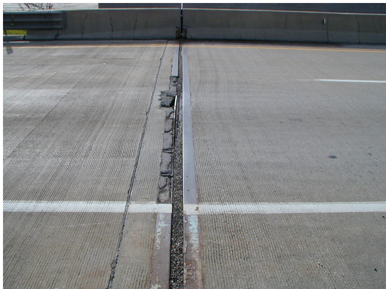
PHOTO #1 12 FOOT OF THE APPROACH SLAB SIDE OF THE DECK ARMOR, WAS CUT OUT IN LANE #2.
