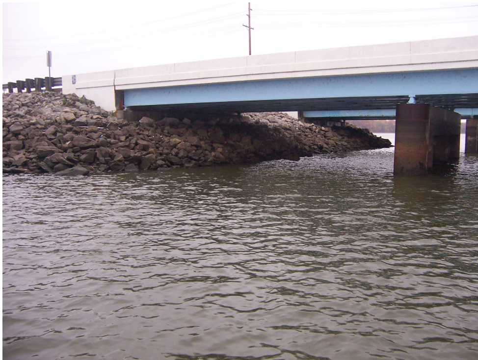
Photo 6 – Facing Southeast. East Abutment with large Riprap Stone Shore Protection.
