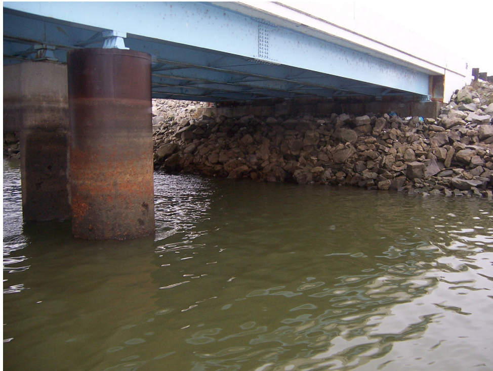
Photo 5 – Facing West. West Abutment with large Riprap Stone Shore Protection.
