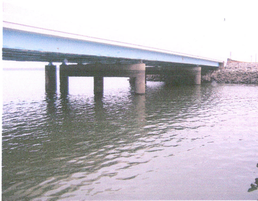
South Elevation View looking East
