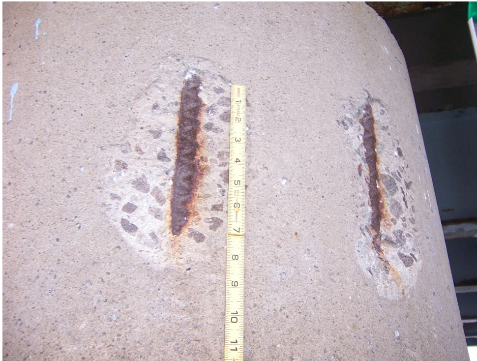
Photo 7 – Facing North. South end of Pier 3 Cap with Spalls and exposed Rebar. (9-inch high x 6-inch wide x 1-inch deep)
