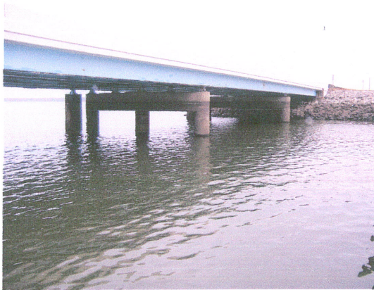
South Elevation View looking East
