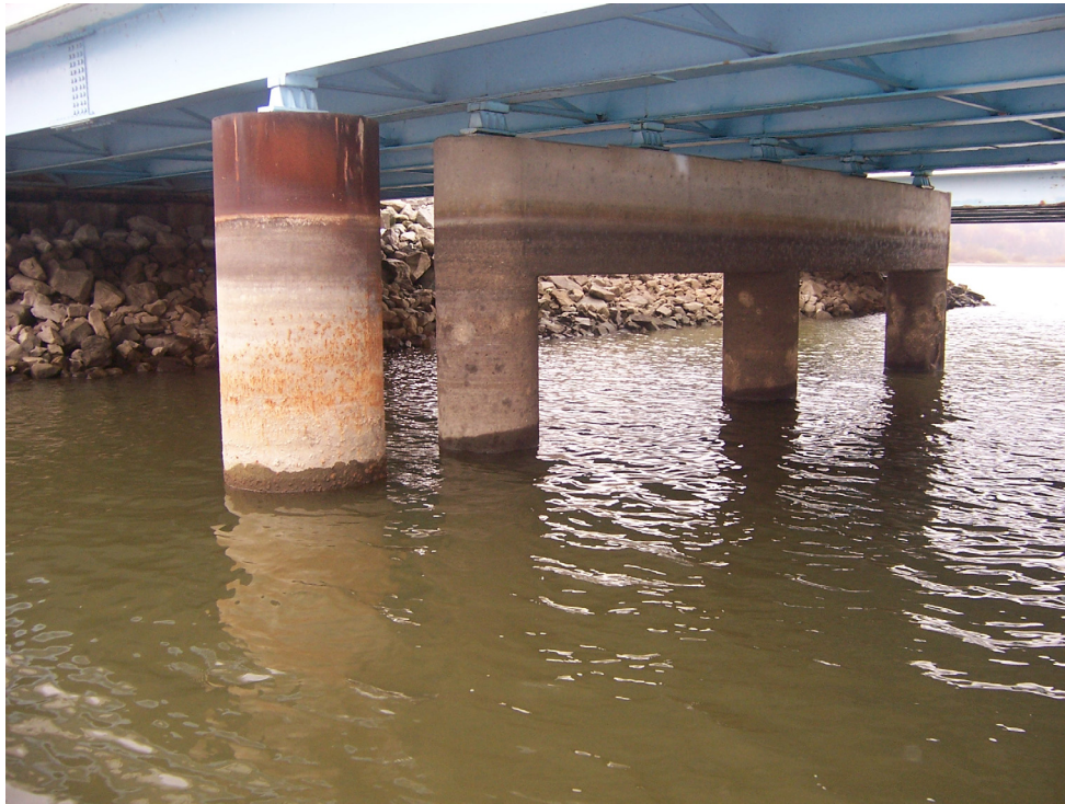
Photo 5 – Facing Northwest. Pier 1 and West Abutment with Riprap Stone.
