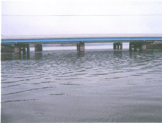
South Elevation View looking North
