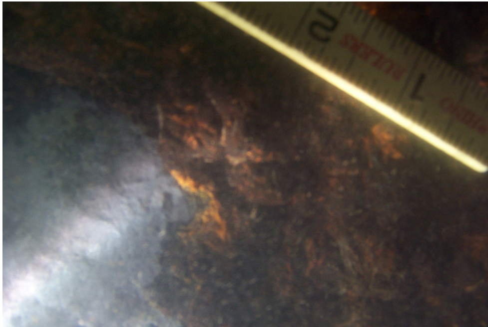
Photo 7 – Facing North. South side of Pier 3 steel jacket on the drilled shaft at the mudline. Typical 1/8-inch thick corrosion of the steel.
