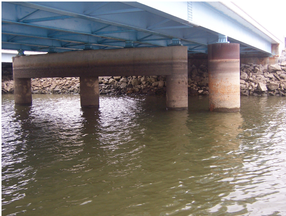
Photo 6 – Facing East. Pier 3 and East Abutment with Riprap Stone.
