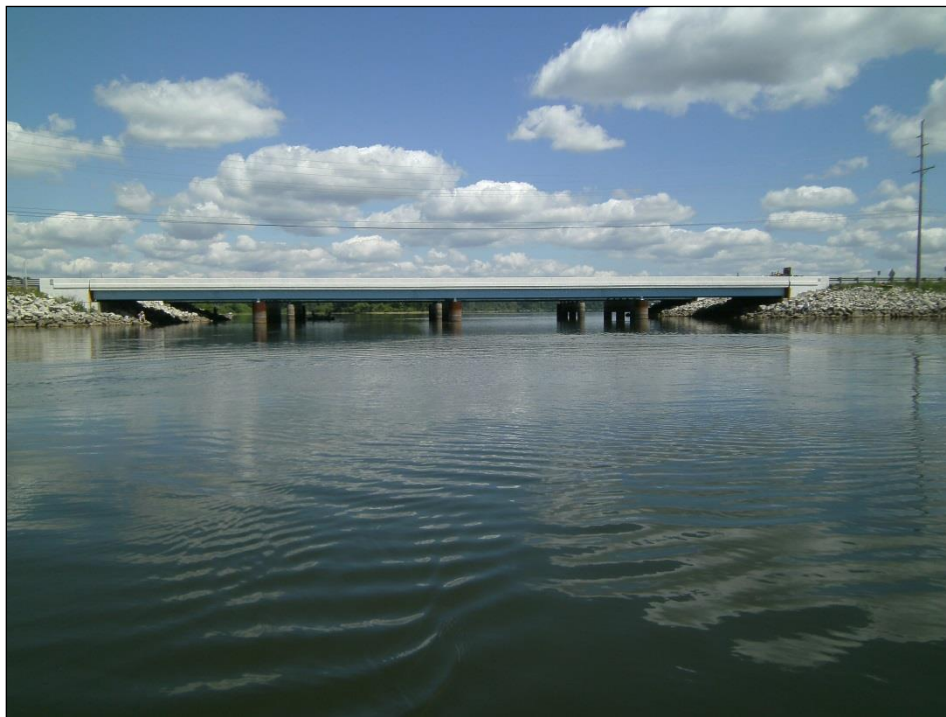
(South Elevation of Bridge)
