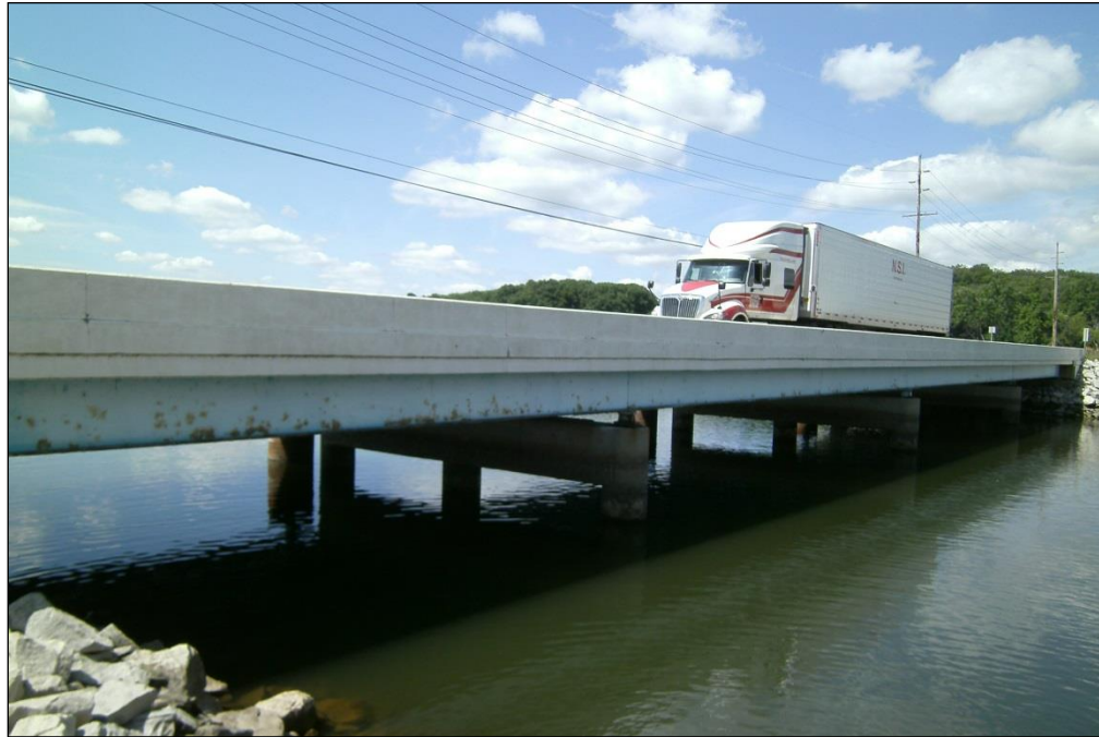
Photograph 1 Overall View of the North Elevation. Looking Southwest
