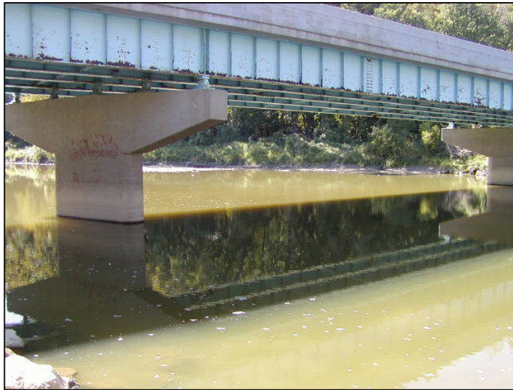
General Elevation View
