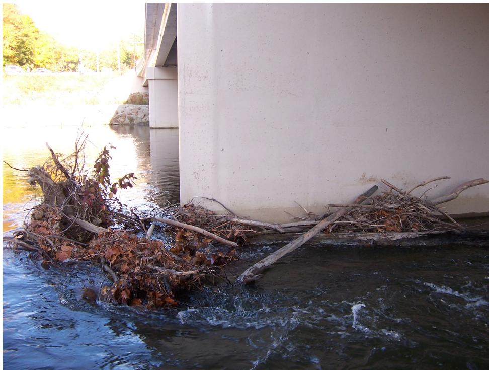
Photo 6 – Facing North. Pier 2 with Timber Debris on the Upstream Nose.
