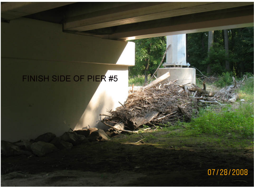
P4: NOTE LOG JAM BETWEEN PIER 5 AND UTIL POLE FOUNDATION. HIGH WATER FLOWS THRU HERE.
