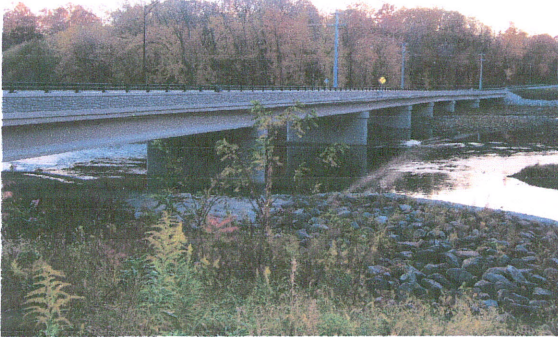
West Elevation of Bridge
