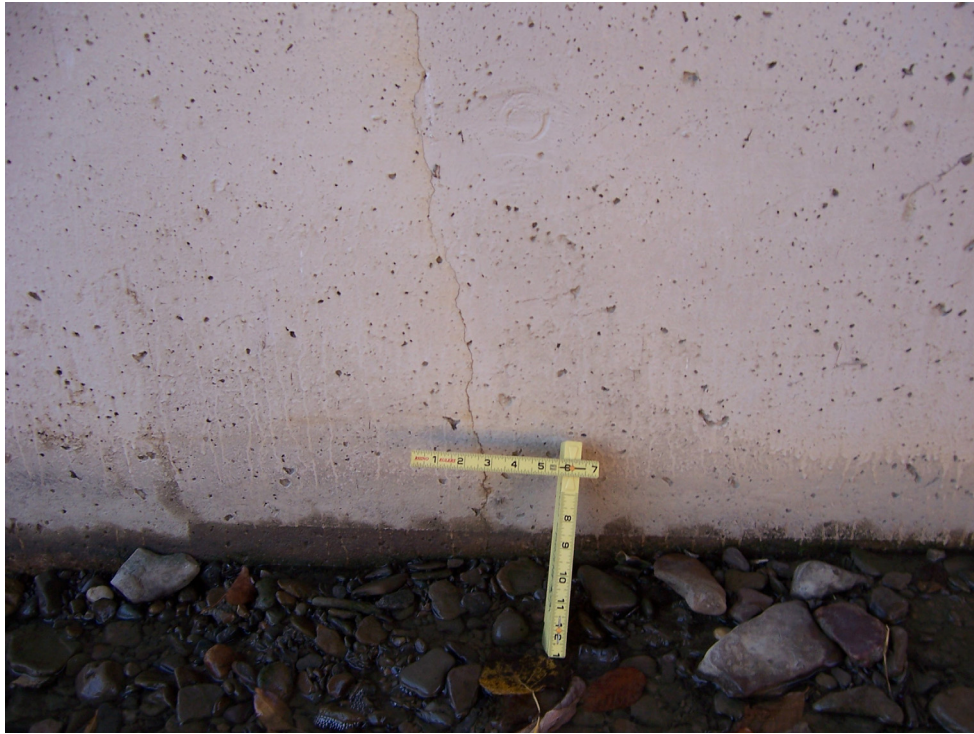
Photo 9 – Facing South. Hairline Vertical Crack at the center of the north face of Pier 2.
