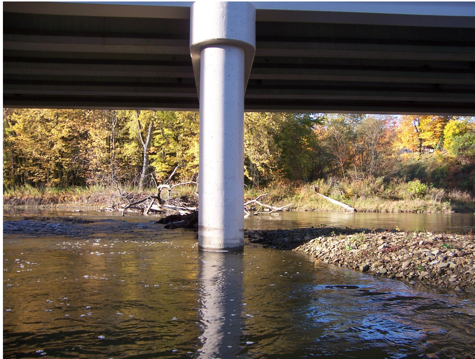
Photo 7 – Facing West. Pier 2 with a pile of stone deposited on the northeast corner.
