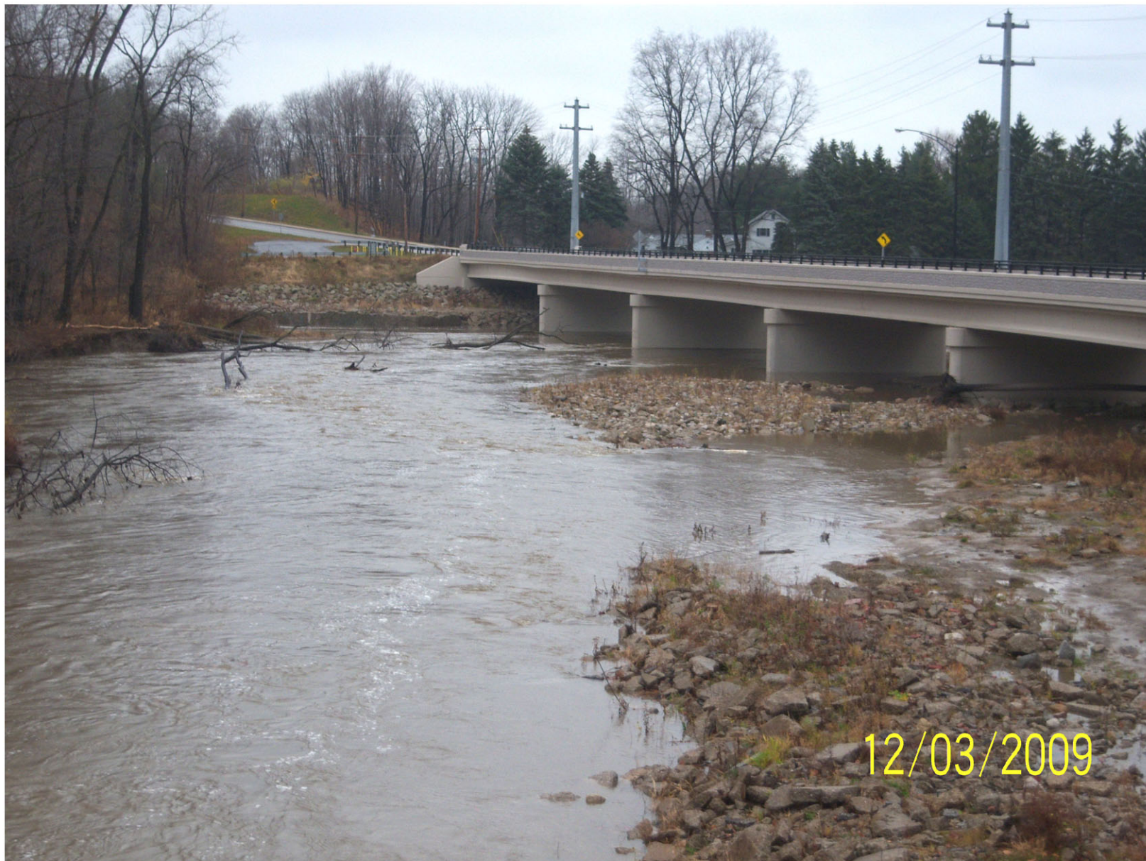
Braided channel upstream of SR 84.JPG
