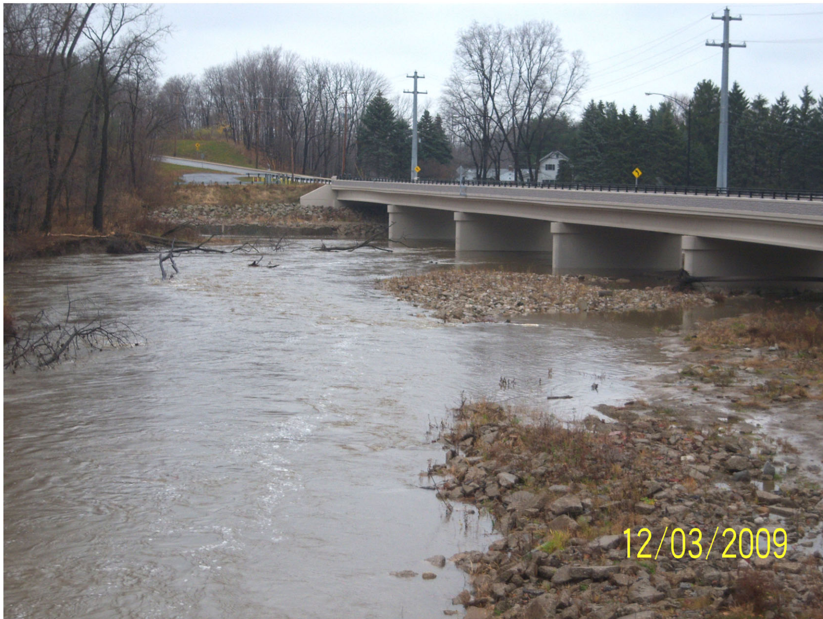
Braided channel upstream of SR 84.JPG
