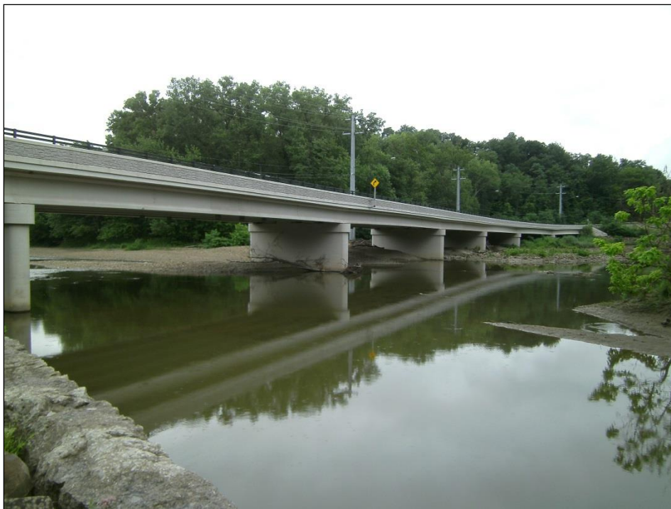
(West Elevation of Bridge)
