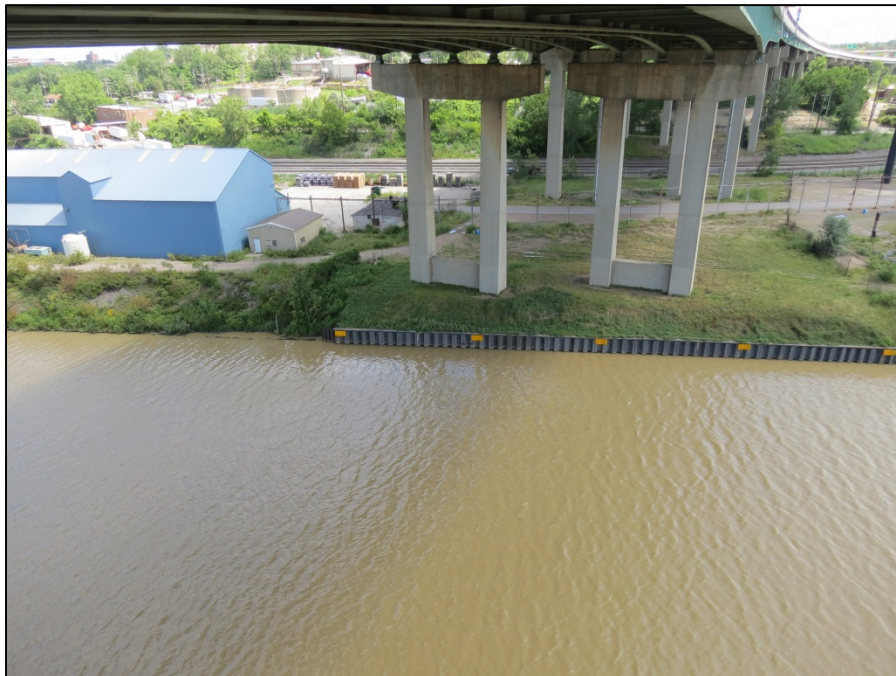
Picture #49: General view of east bank bulkhead, looking east.
