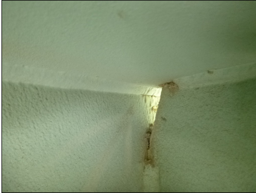
Picture #30: Possible crack or weld undercut on girder G in span 9R, looking south.
