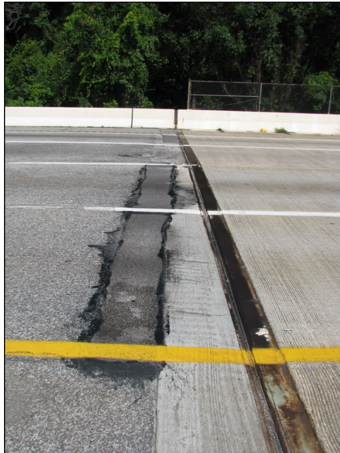
Picture #7: Rear abutment expansion joint header repair, looking north.
