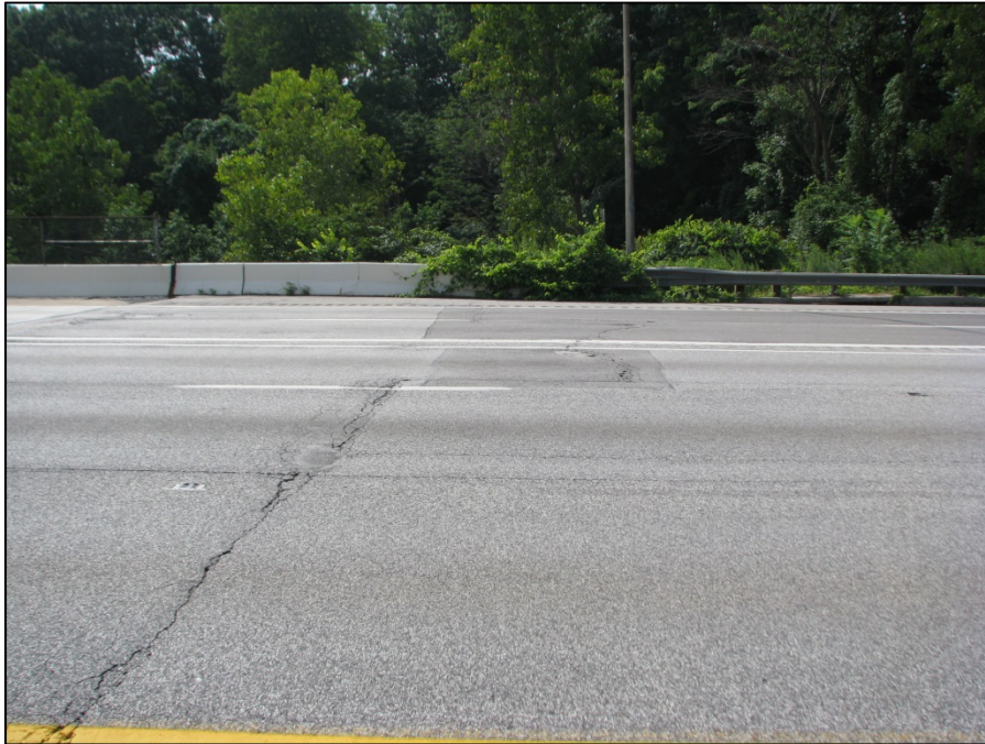
Picture #1: Rear approach wearing surface looking south.
