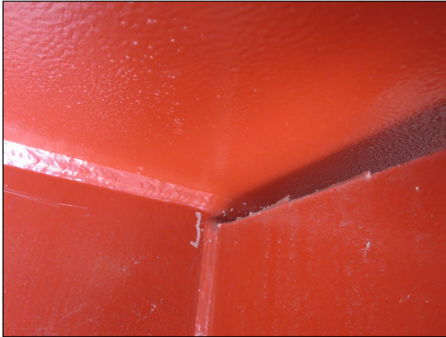
Picture #12: New 1.75” active crack on south face of girder G, span 7.
