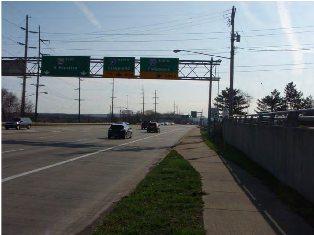
Photo 24. S.R. 82 and I-71S south side, looking east
