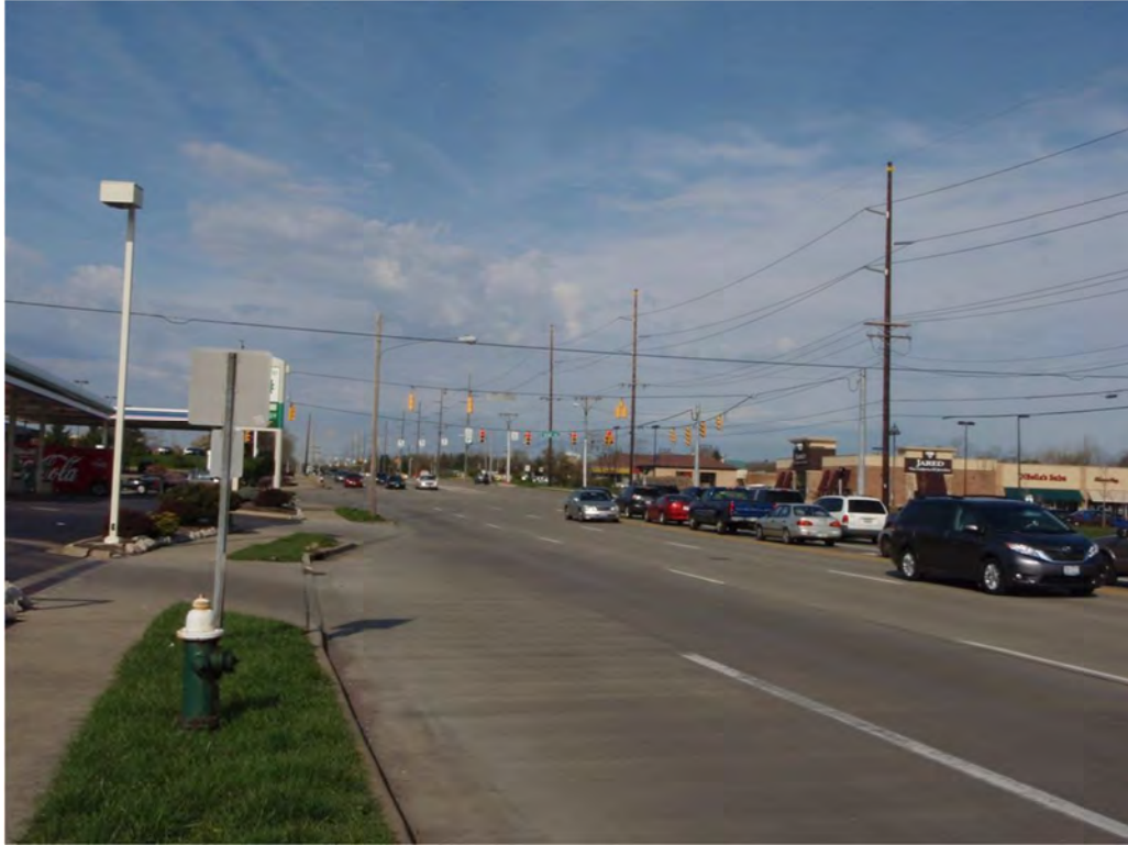
Photo 17. S.R. 82 and Howe Rd. south side, looking west
