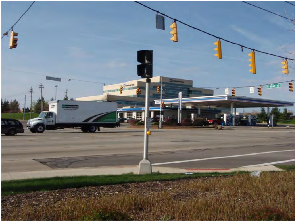
Photo 10. S.R. 82 and Howe Rd. rotated pedestrian head
