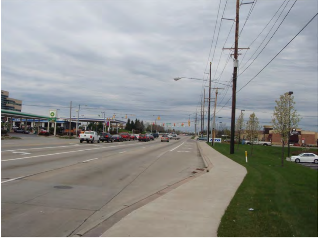
Photo 13. S.R. 82 and Howe Rd. north side, looking west
