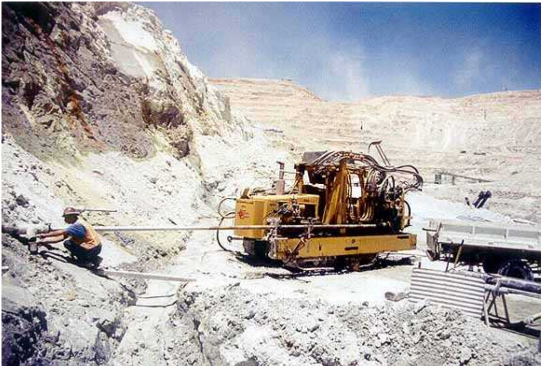
Figure 8.2: Pictures of horizontal drain installation equipment
