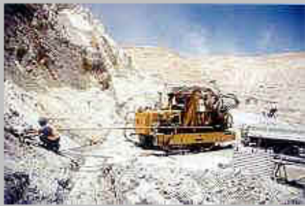
Horizontal Drilling in Chile
