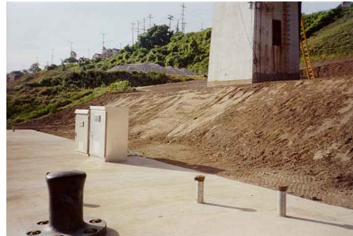
Figure 5.19 Photo showing the construction of the tie beams and the buildup of fill on top
