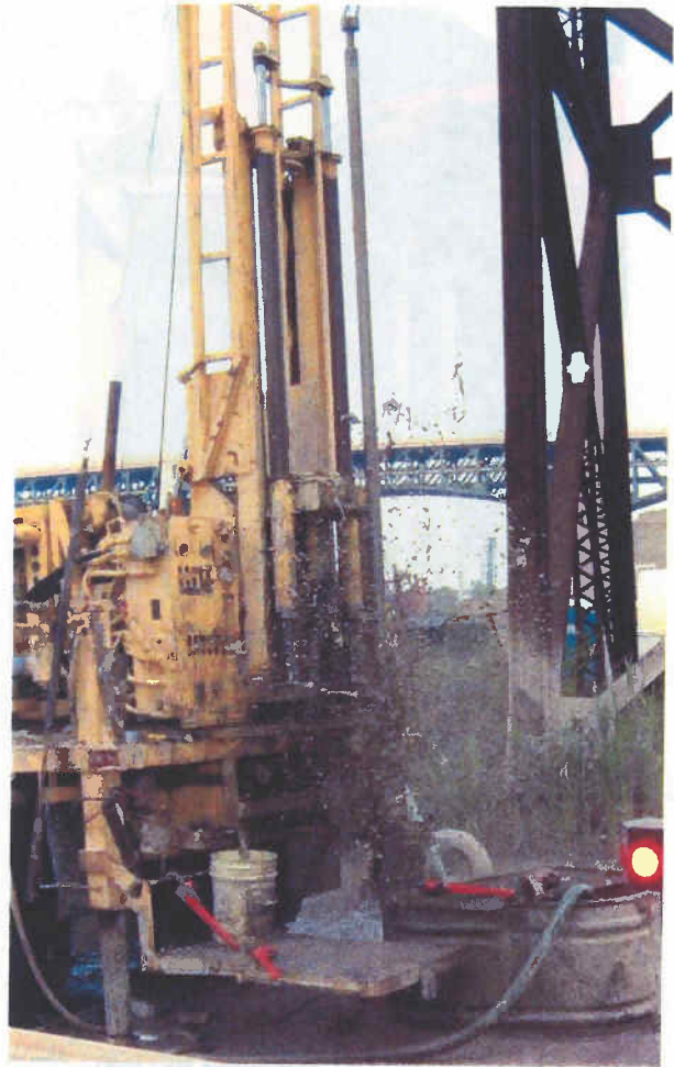
b) Water/gas erupting during drilling operations at B-05-15.
