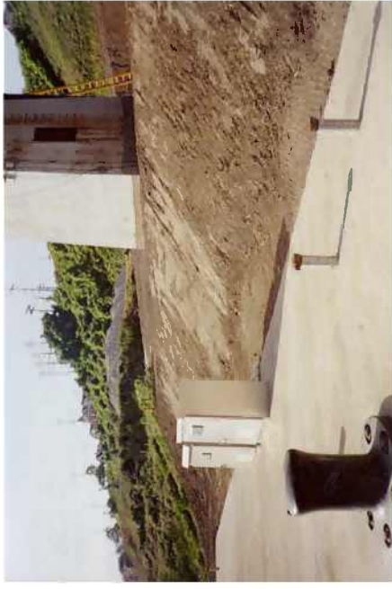
Figure 5.19 Photo showing the construction of the tie beams and the buildup of fill on top
