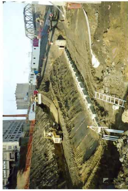
Figure 5.19 Photo showing the construction of the tie beams and the buildup of fill on top
