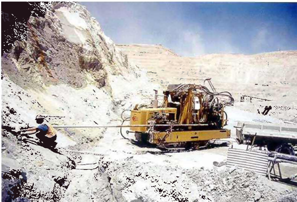
Figure 8.2: Pictures of horizontal drain installation equipment
