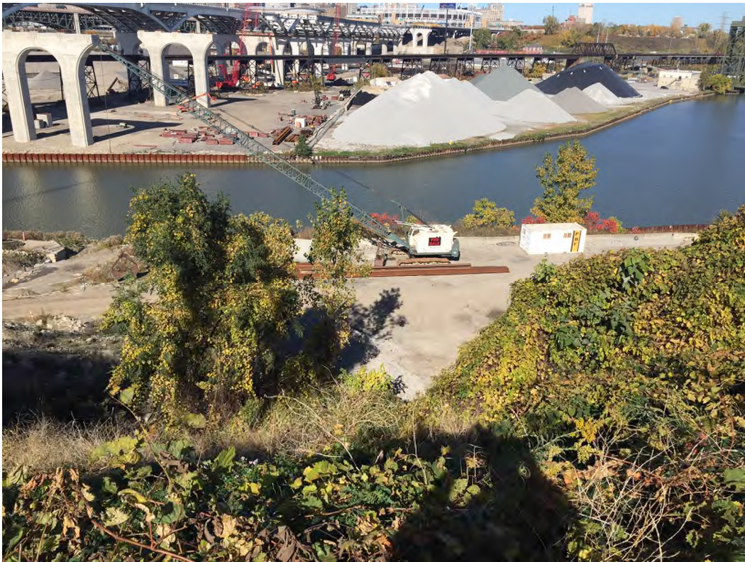
Figure 5. Aggregate stockpile near ODOT's east right-of-way fence (October 23, 2015)
