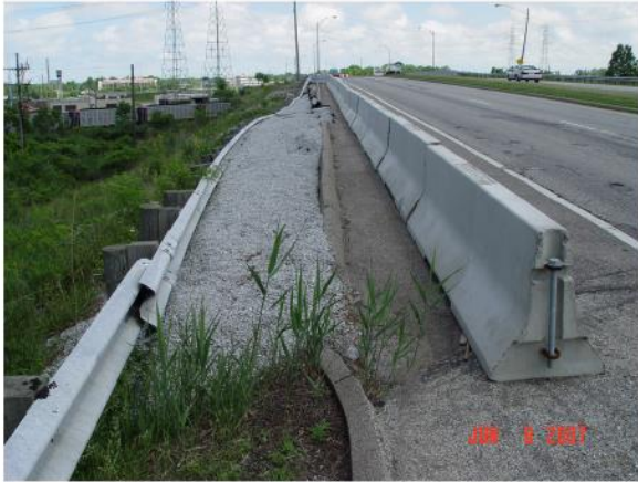
Start-left embankment failure .jpg
