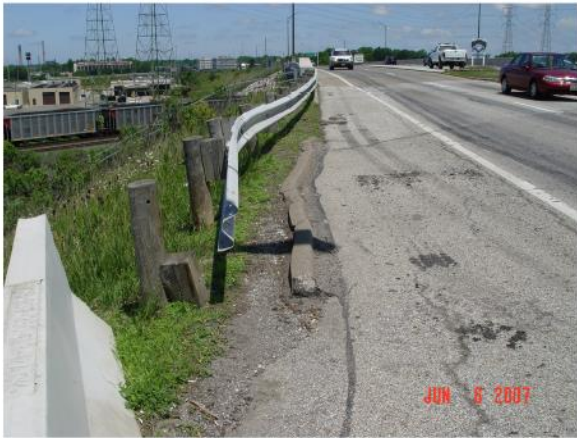
Start-left embankment failure .jpg
