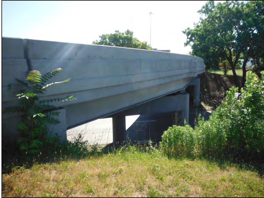
Photo 1: View looking east along the south parapet.
