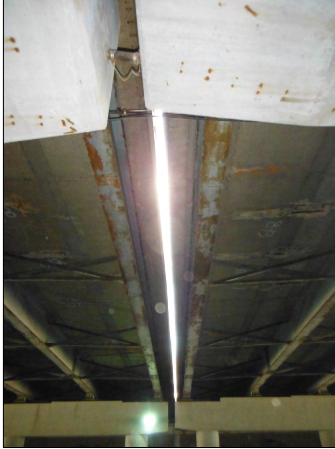
Photo 3: Looking at open center median joint between east and westbound superstructures.
