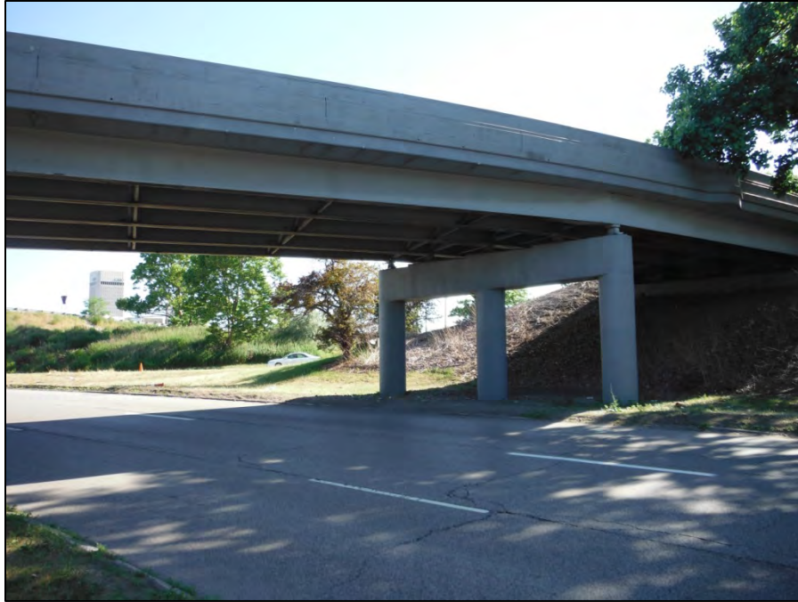
Photo 4: Looking north at the three lanes under the bridge.
