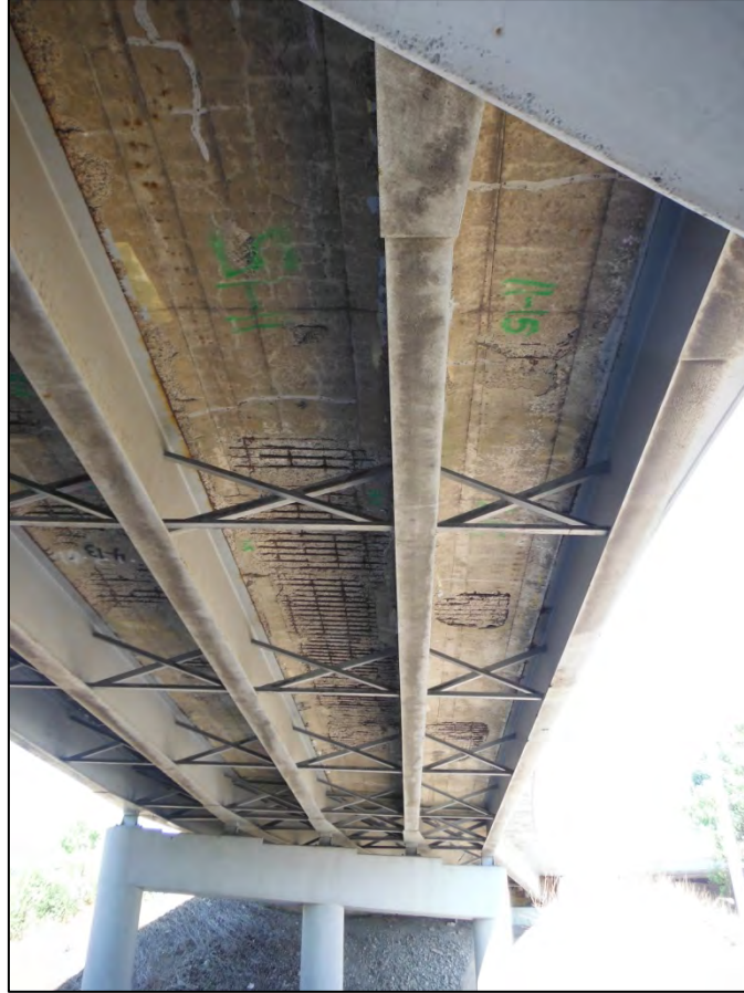
Photo 3: Looking west over traffic lanes.
