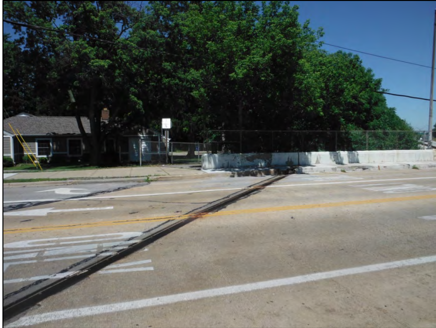
Photo 1: View of north fence and railing at west joint.
