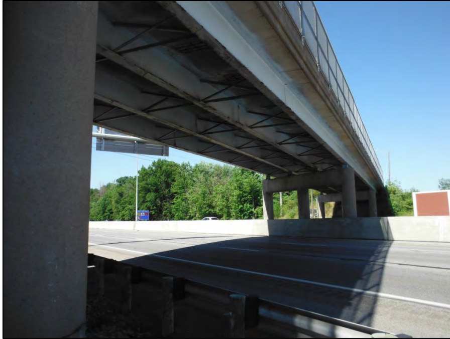
Photo 1: Typical view under the bridge looking north across the eastbound lanes.
