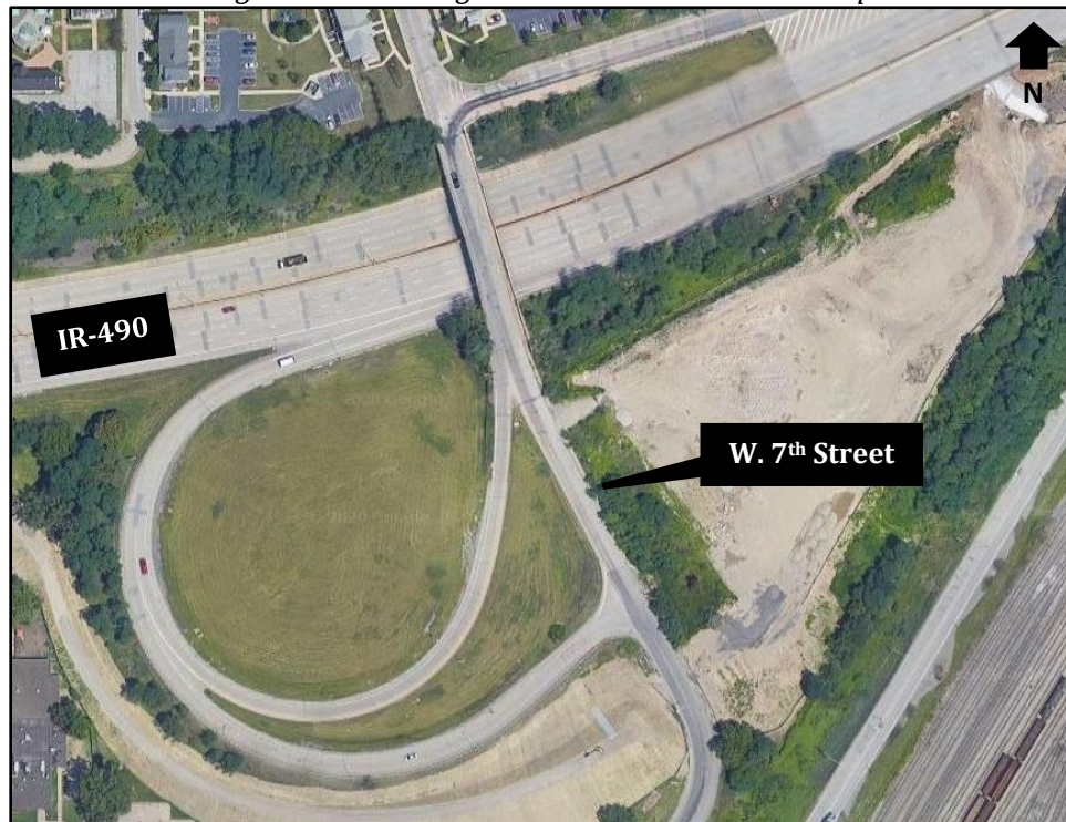
Figure 11 - Existing W. 7th Street Entrance Ramp
