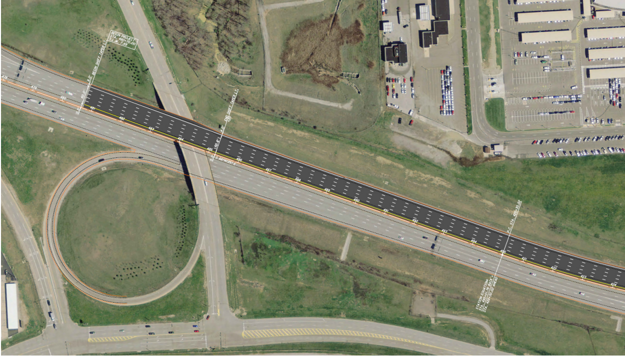
Figure 1. West end of the project, Grayton Rd. exit becomes a drop lane.
