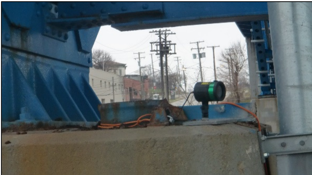
Photo 69 – Private Light Mounted on Top of Pier 2 South.
