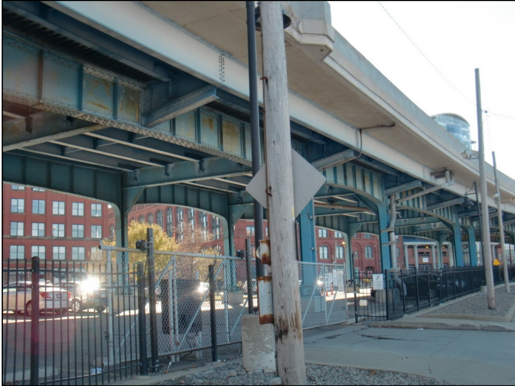
Photo 2 – South Elevation, East Approach – Lakefront Trestle.
