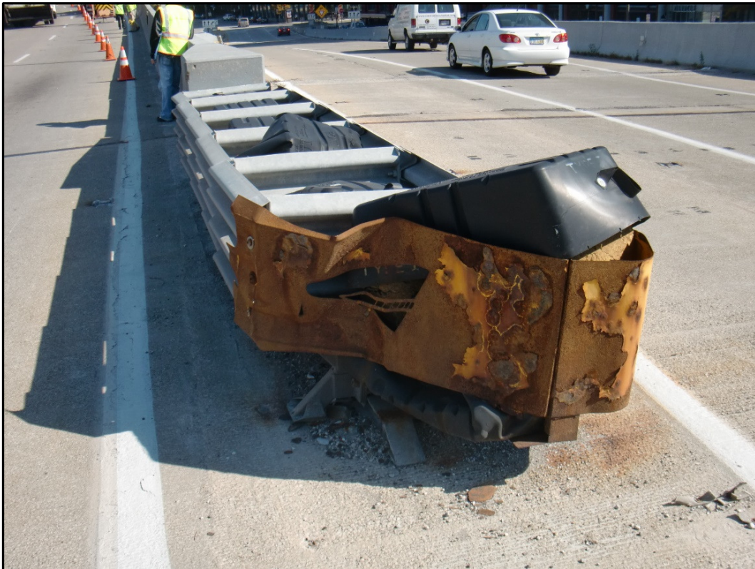
Photo 14 – Damaged Impact Attenuator, Lakeside Ramp - East Approach. (Note: Attenuator was repaired after inspection.)
