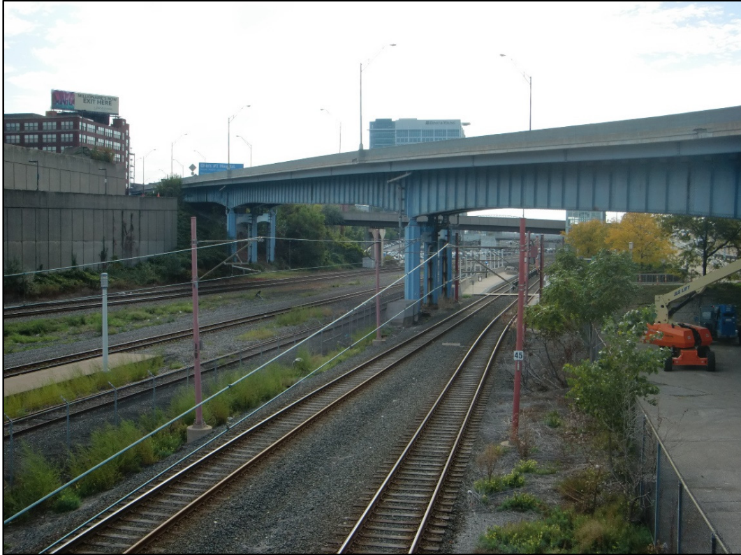
Photo 4 – South Elevation, East Approach – Lakefront Ramp.
