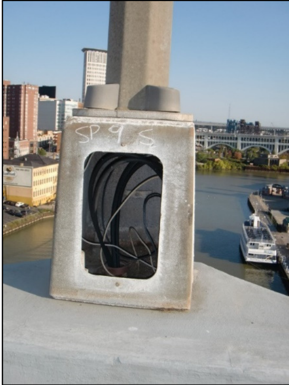
Photo 22 – Open Pull Box, South Railing, Span 9.
