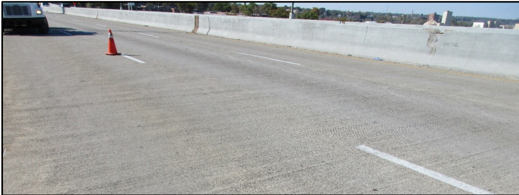
Photo 5 – Typical Good Condition of Slab.
