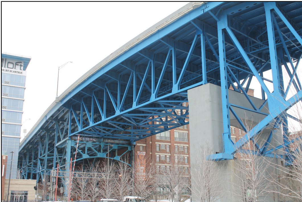
Photo 3 – North Elevation, East Approach – Forward Section.
