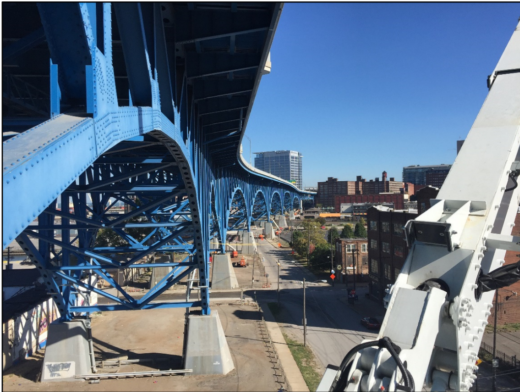
Photo 1 – South Elevation, Main Truss Spans.
