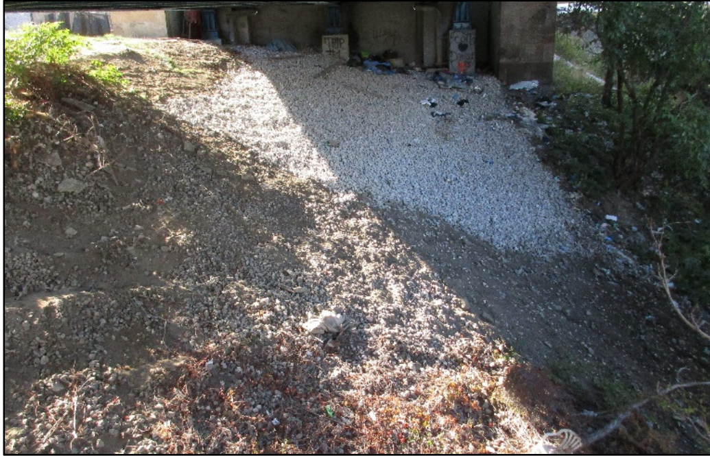
Photo 61 – Slope Protection Repair, East Side of Pier 37.
