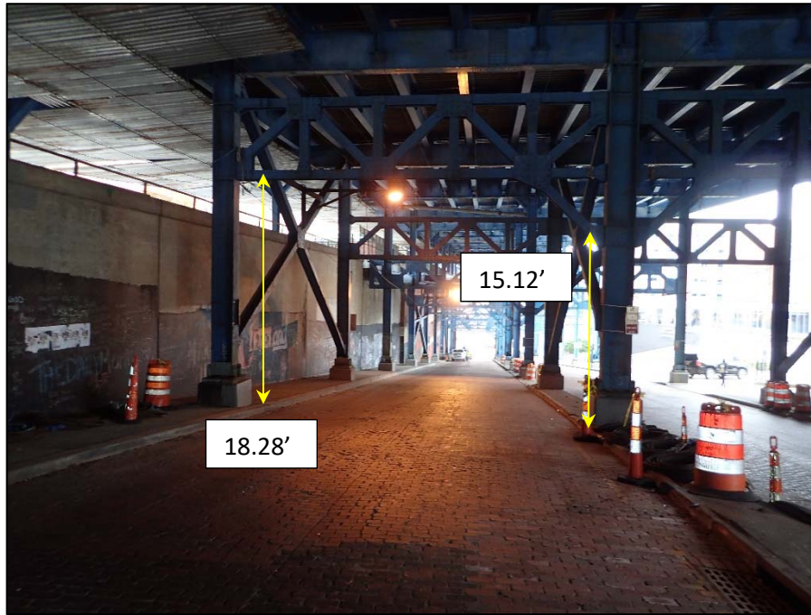
Unit III; Main Avenue, Bent 9, Looking West
