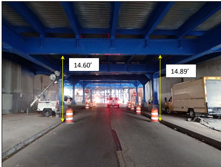
Unit III; Lakeside Avenue Between Bents 14 – 15, Looking West
