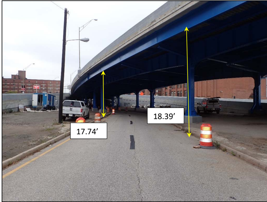
Unit IV; Lakeside Avenue, Westbound, Looking North
