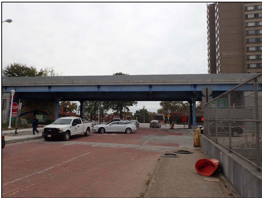
Unit I: Section C, South elevation
