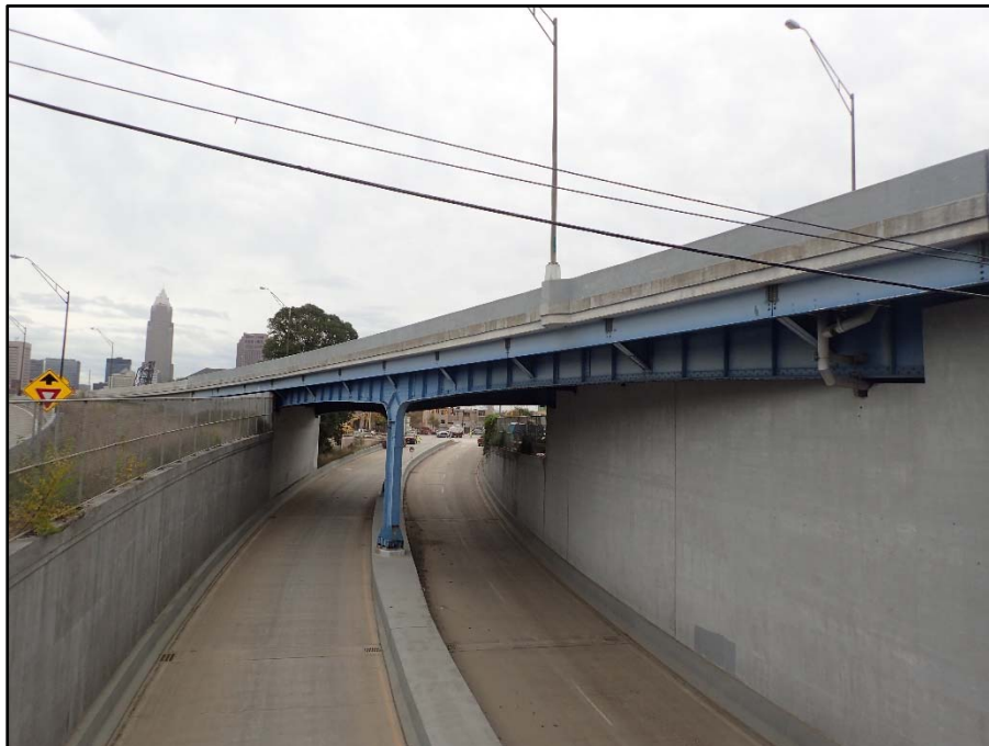
Unit I: Section M, North elevation
