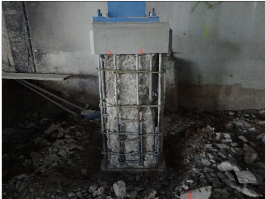
Photo 38 – Unit I, Section N, Frame 8; Active rehabilitation of frame base
