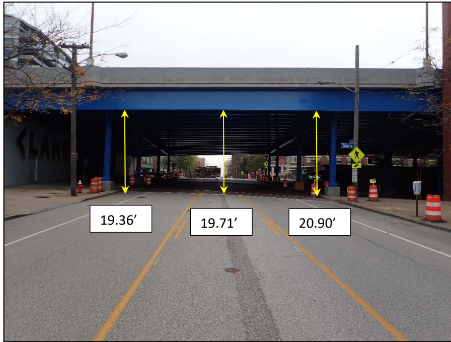
Unit III; West 9 th Street, North fascia, Looking South
