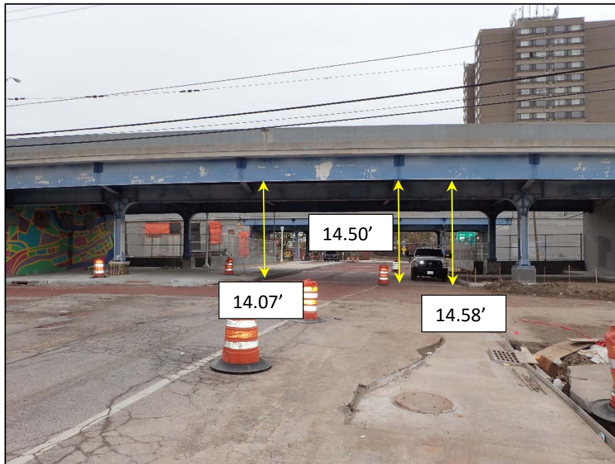
Unit I, Section K; West 28 th St. Eastbound lanes, Looking North
