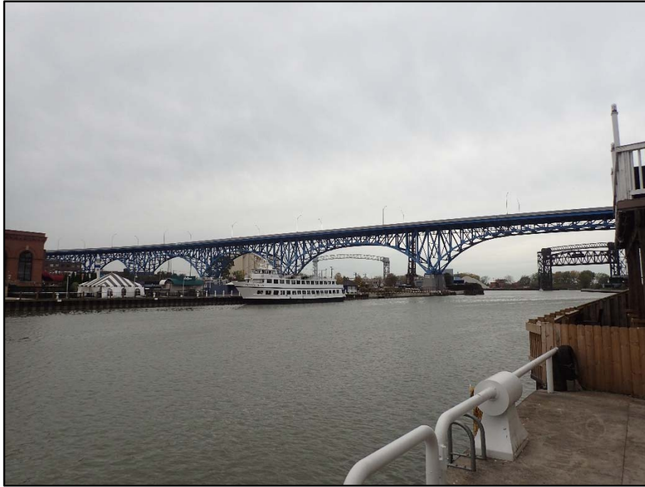
Unit II: Main Truss Spans, South elevation
