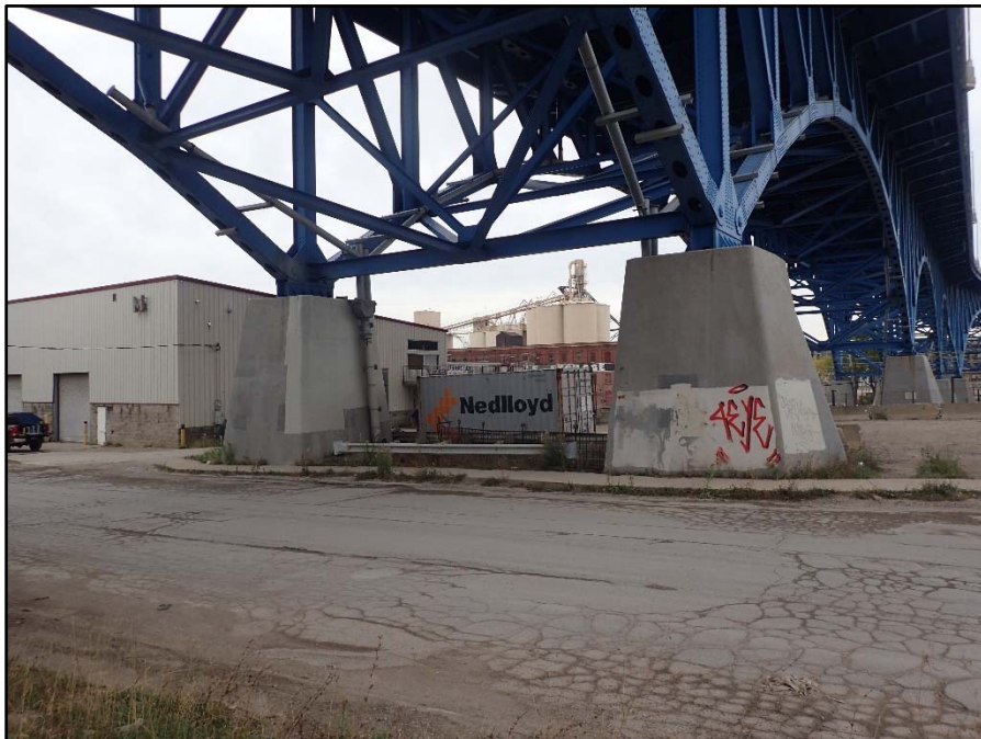
Unit II: Main Span Truss, Typical pier
