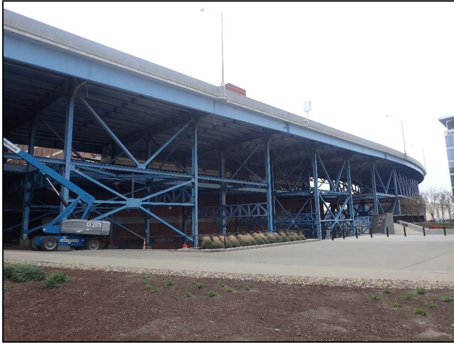
Unit III: East Approach, Forward Section, North elevation
