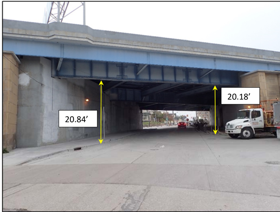
Unit I, Section N; West 25 th Street, North fascia, Looking South
