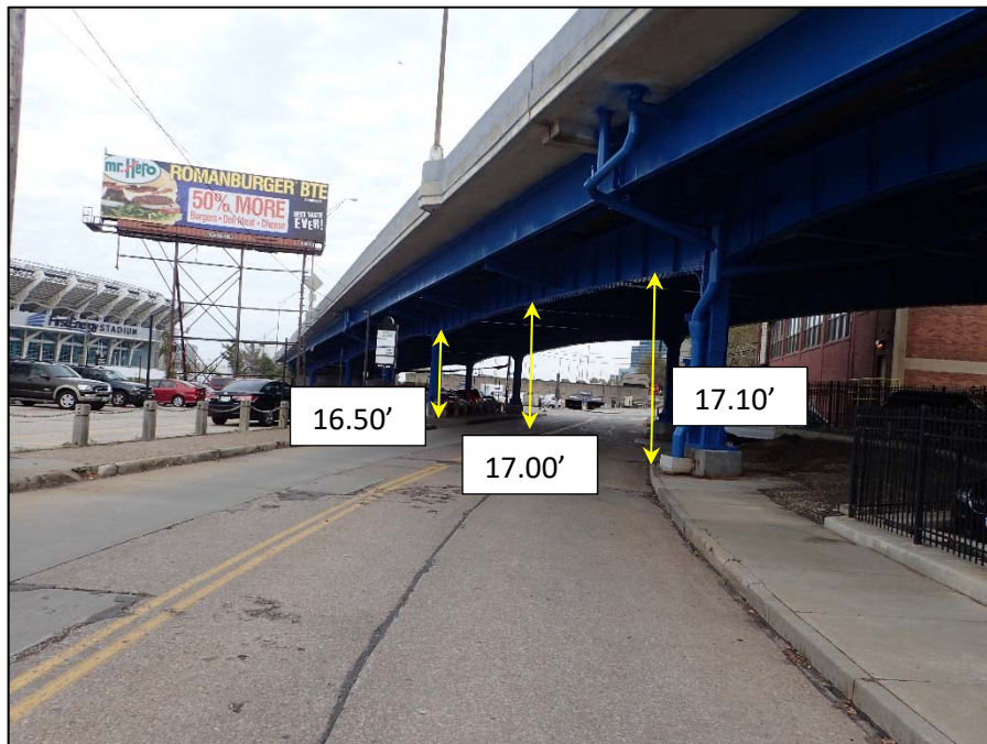
Unit IV: Summit Avenue, Looking East
