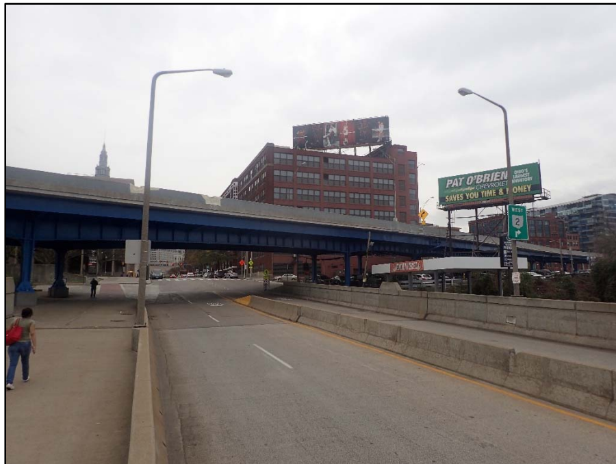
Unit IV: East Approach, Lakefront Trestle; North elevation
