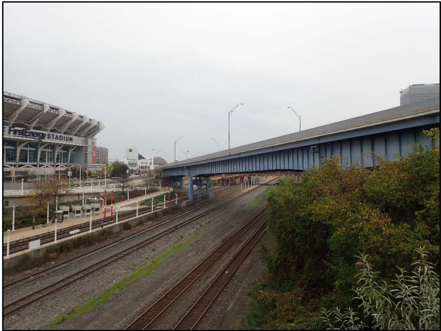
Unit V: East Approach, Lakefront Ramp Section; North elevation
