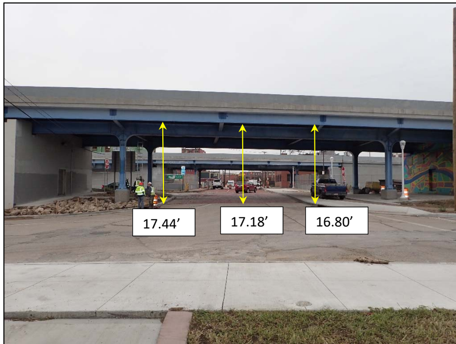
Unit I, Section C; West 28 th Street, Westbound lanes, Looking South
