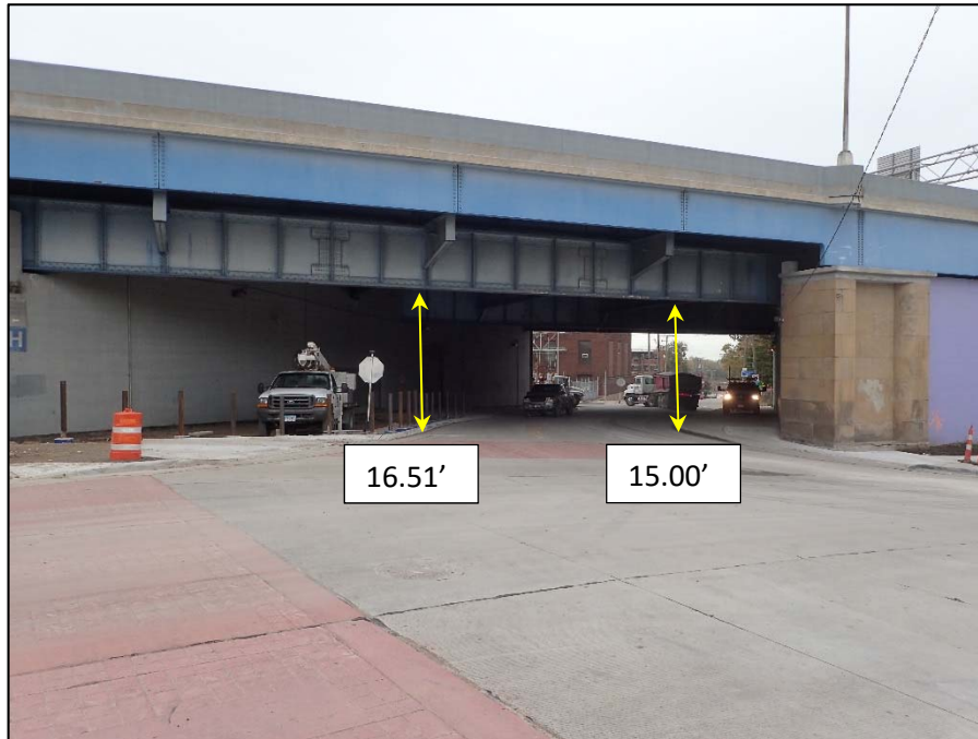
Unit I, Section N; West 25 th Street, South fascia, Looking North
