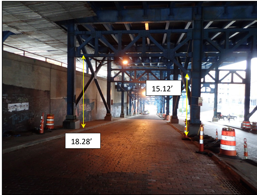
Unit III; Main Avenue, Bent 9, Looking West
