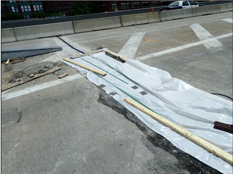
Photo 5 - Section IV, Joint C; Joint being replaced
