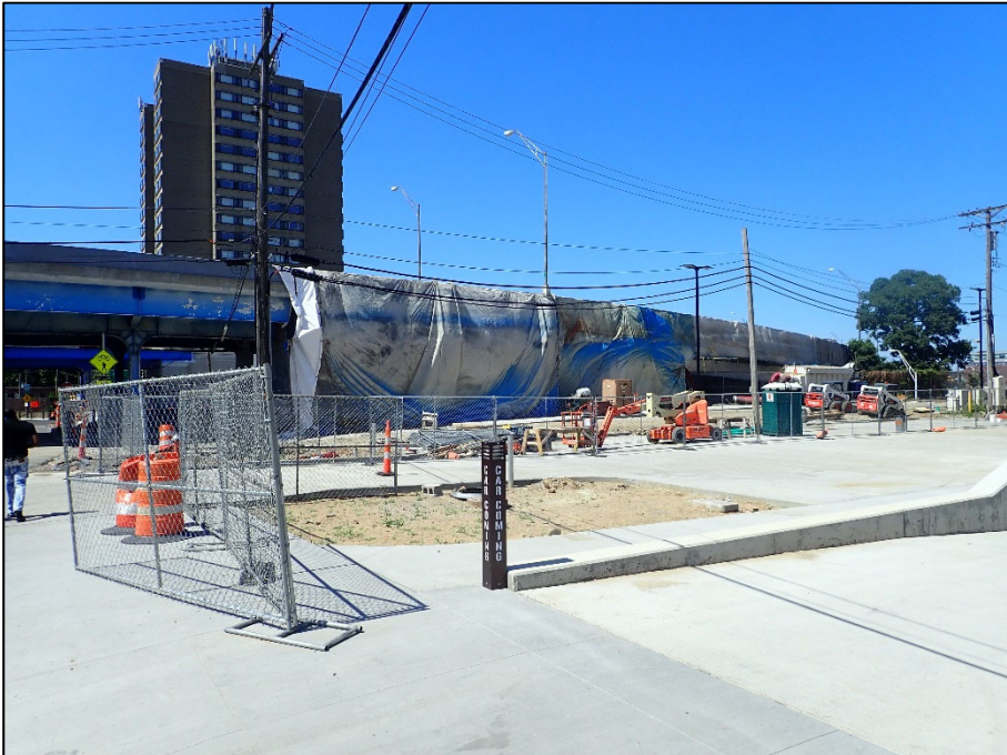
Photo II: Unit I: Section K, South elevation; tarped for painting
