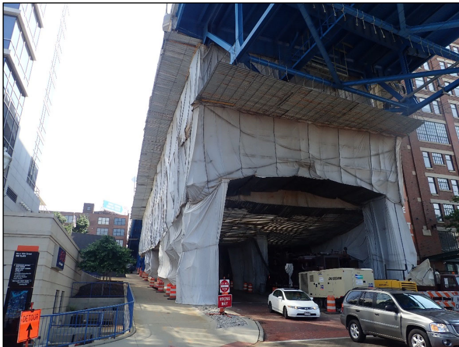
Photo VIII: Unit III: East Approach, Forward Section; Ongoing painting
