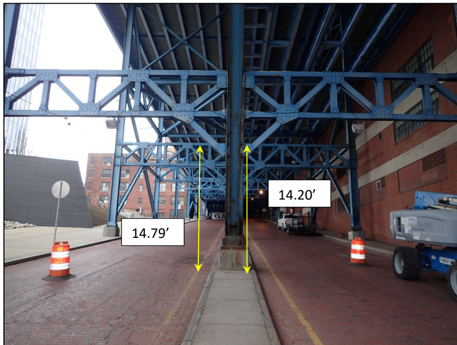
Unit III, Frame & Braced Column Section; Main Avenue, Looking East below Trestle
