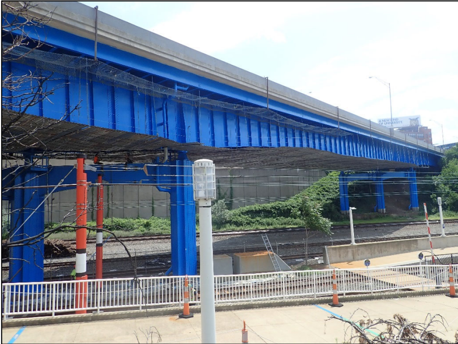
Photo X: Unit V: East Approach, Lakefront Ramp Section; Ongoing painting
