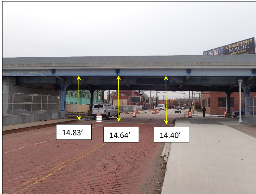
Unit I, Section K; West 28 th St., Eastbound lanes, Looking South
