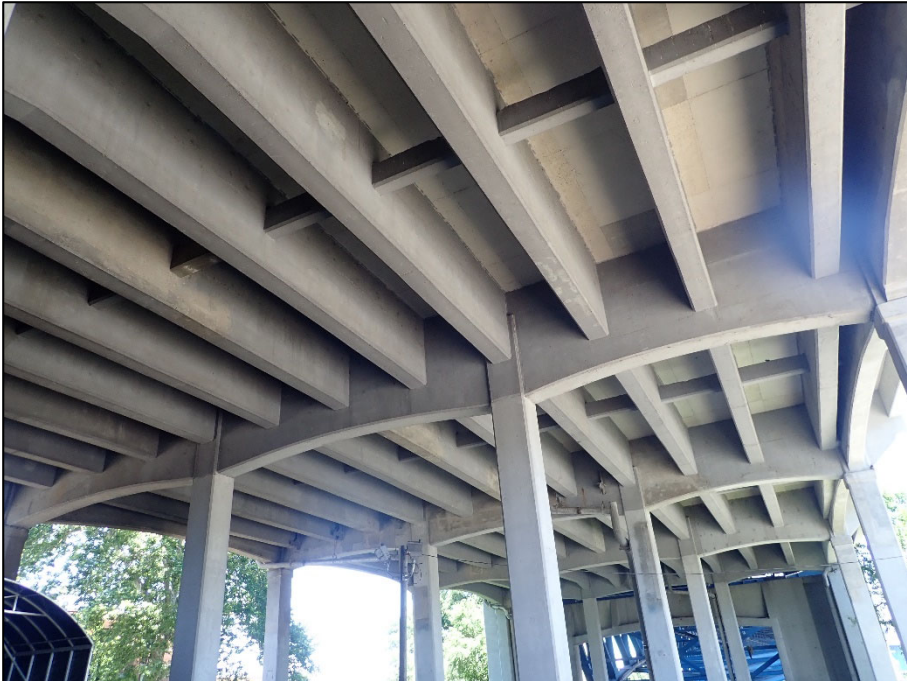
Photo V: Unit I: Section P, Superstructure
