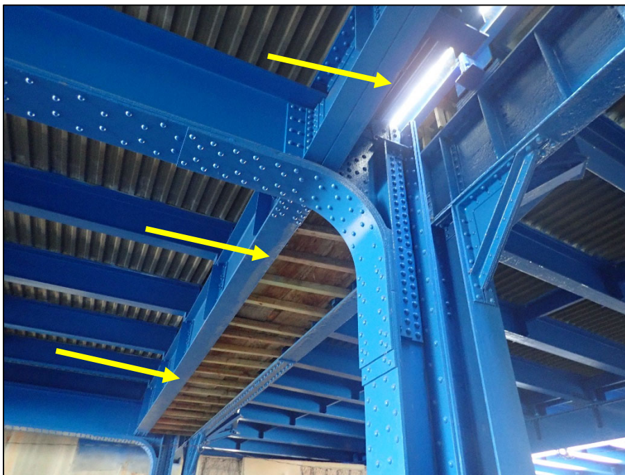
Photo 4 – Section IV, Joint C; Joint being replaced
