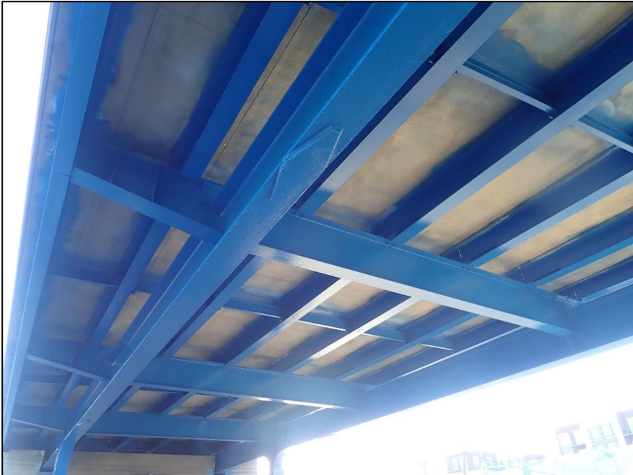
Photo I: Unit I: Section C, Superstructure cleaned and painted
