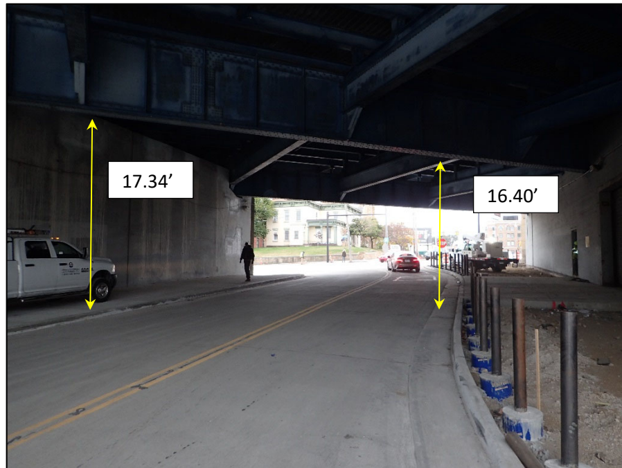
Unit I, Section N; West 25 th Street, Center Girder, Looking South
