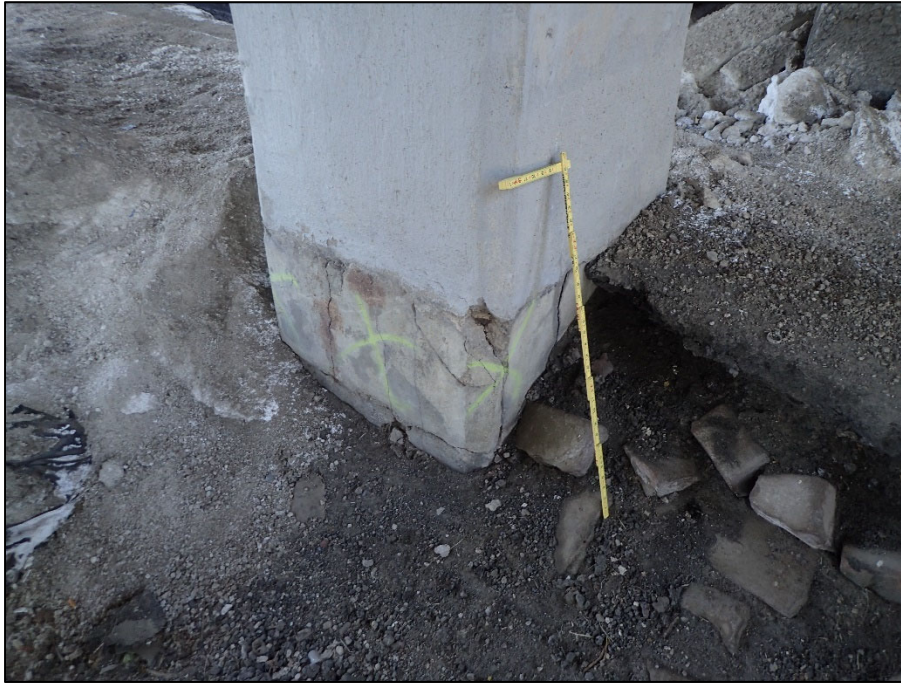
Photo 13 – Unit I, Section P, Pier 2; base of column marked for repair
