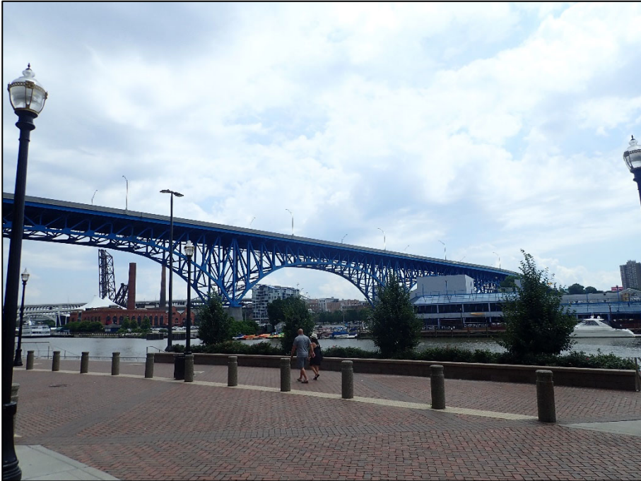
Photo VI: Unit II: Main Truss Spans, South elevation
