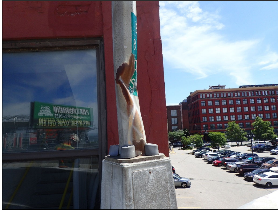
Photo 1 – Joint B2, East parapet; damaged light post
