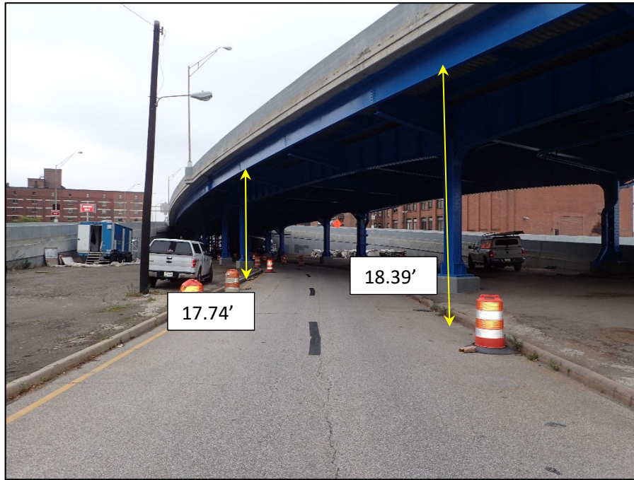
Unit IV; Lakeside Avenue, Westbound, Looking North
