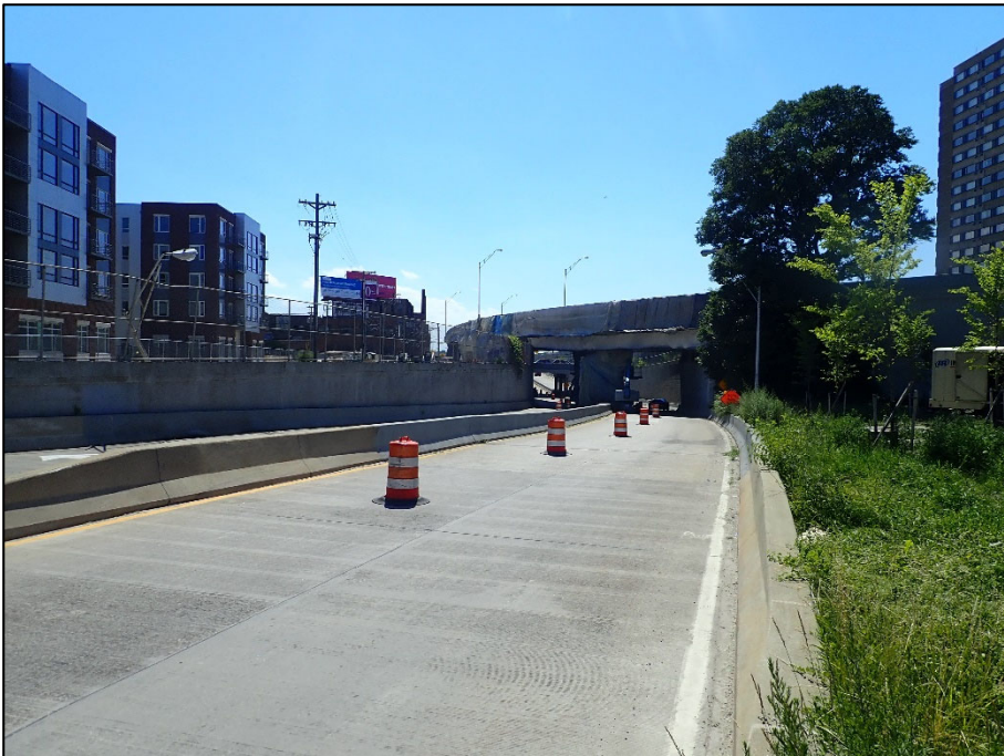
Photo III: Unit I: Section M, North elevation; tarped for painting
