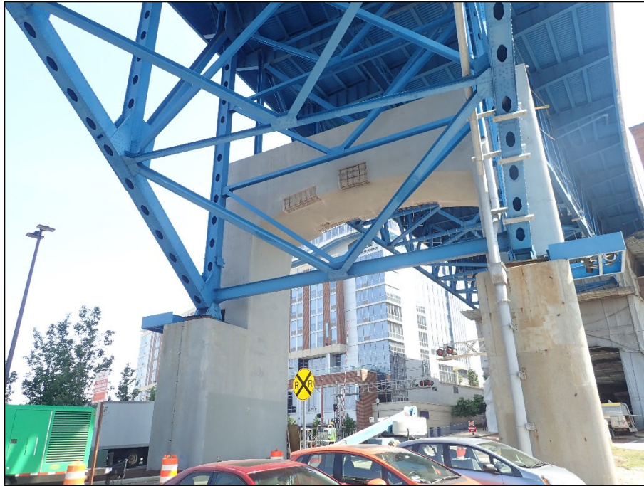
Photo VII: Unit II: Main Span Truss, Typical pier; Ongoing rehab work
