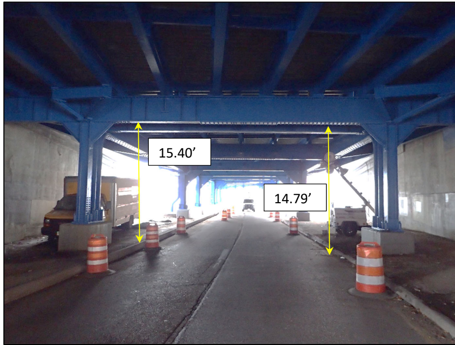
Unit III; Lakeside Avenue, Bent 14, Looking East
