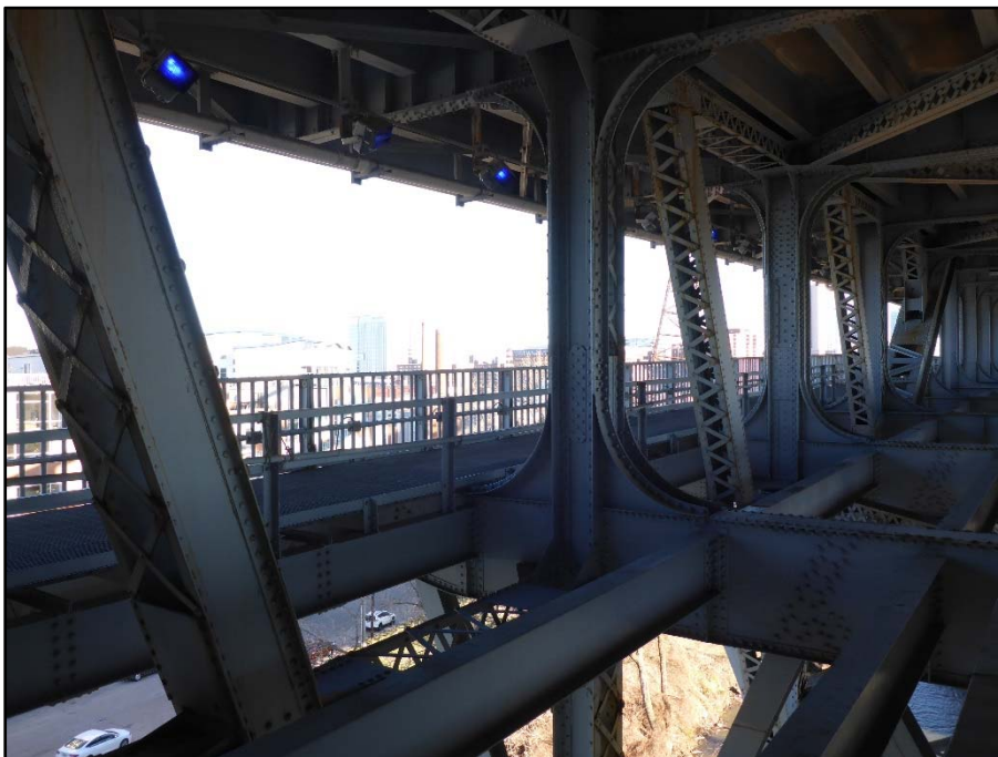
Photo 27 – Typical truss condition
