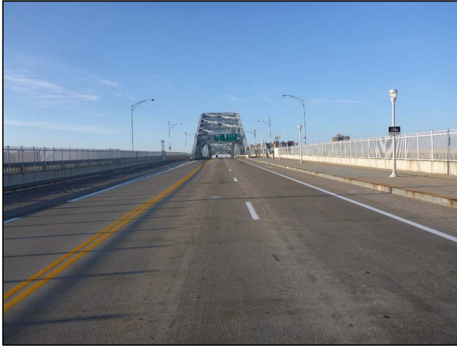
East end view looking West
