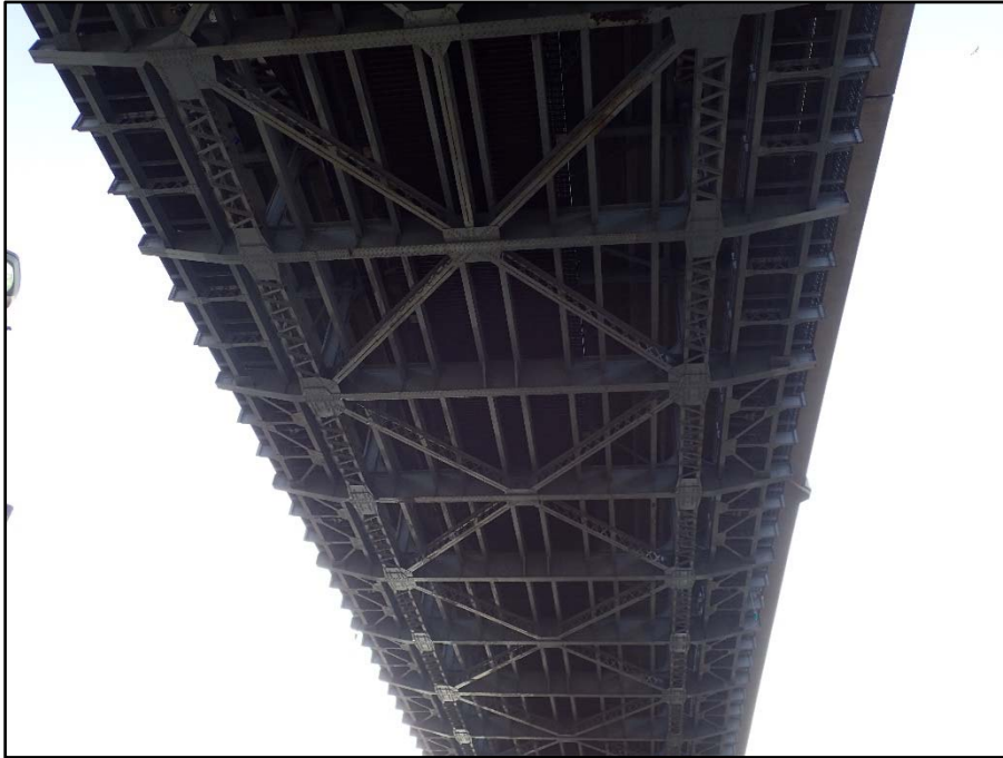
Photo 26 – Typical superstructure condition
