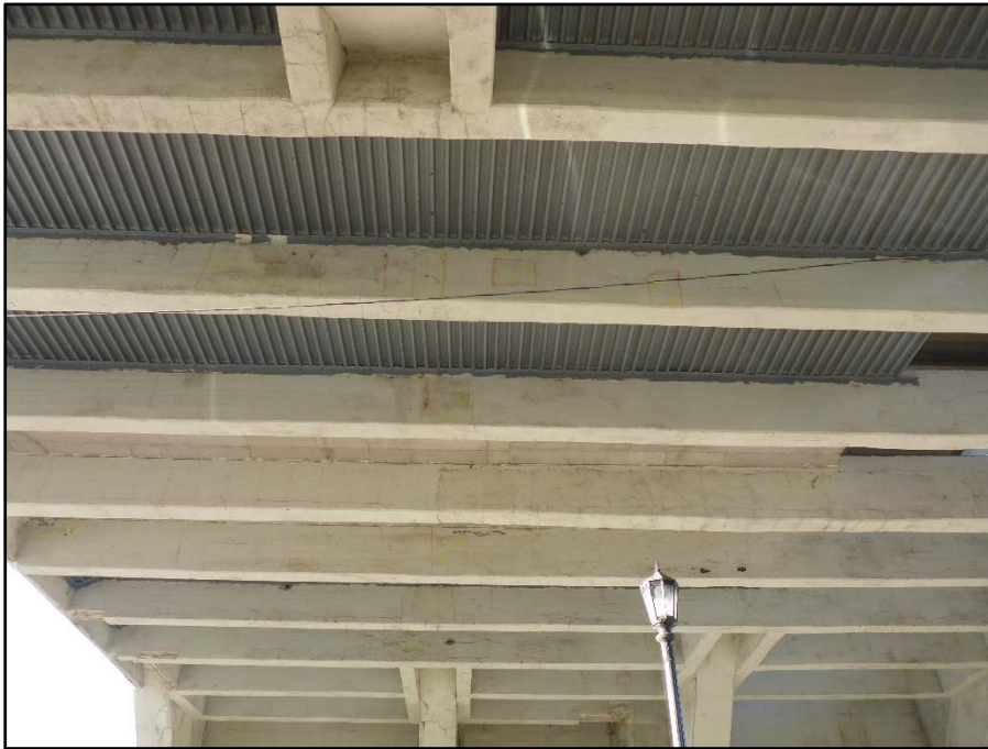
Photo 1 – Typical lower deck soffit West Approach
