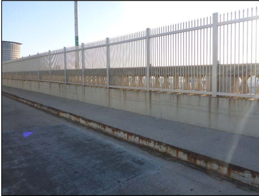
Photo 5 – Typical bridge rail condition
