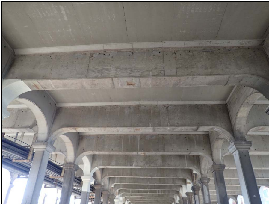
Photo 2 – Typical upper deck soffit Span 2
