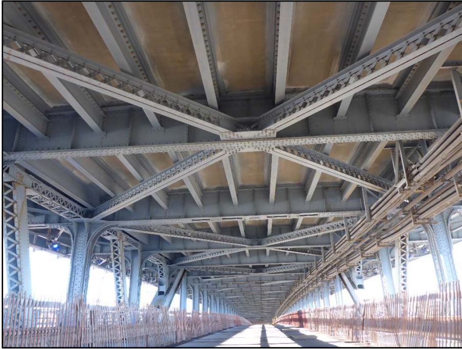
Photo 3 – Typical upper deck soffit Span 4
