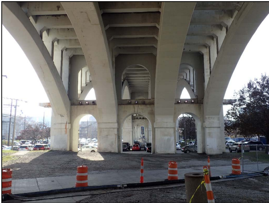
Photo 37 – Pier typical condition
