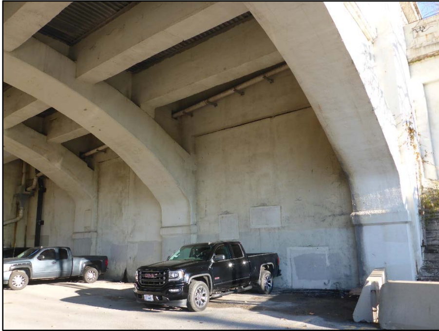
Photo 36 – East Abutment typical condition
