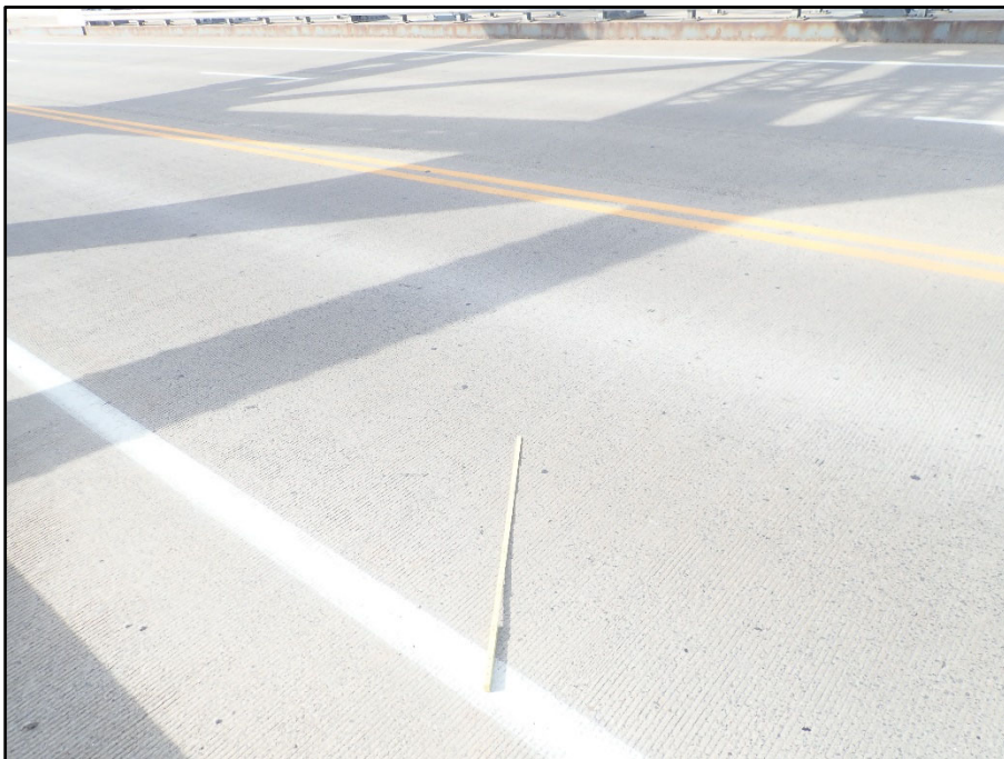
Photo 4 – Typical upper deck wearing surface condition
