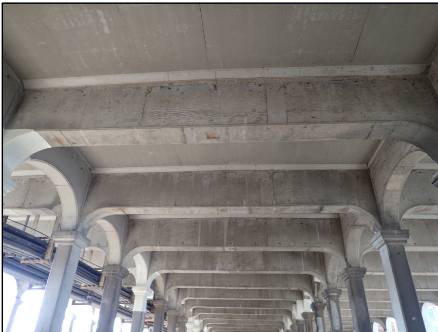
Photo 2 – Typical upper deck soffit Span 2
