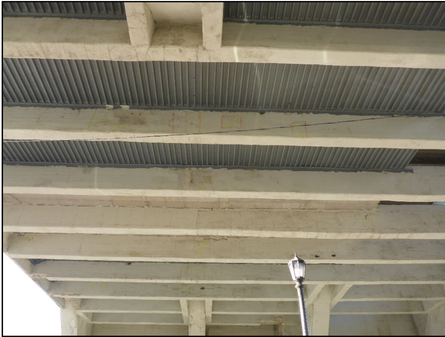
Photo 1 – Typical lower deck soffit West Approach
