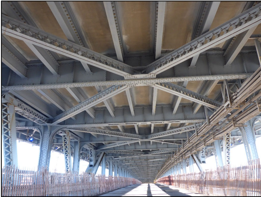
Photo 3 – Typical upper deck soffit Span 4
