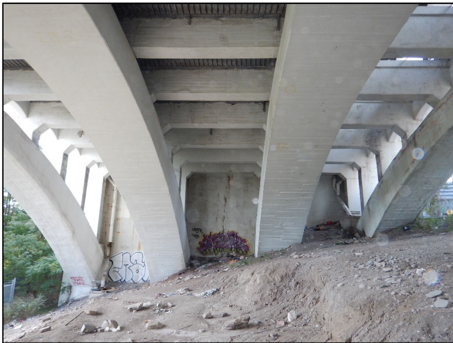
Photo 37 – West Abutment typical condition
