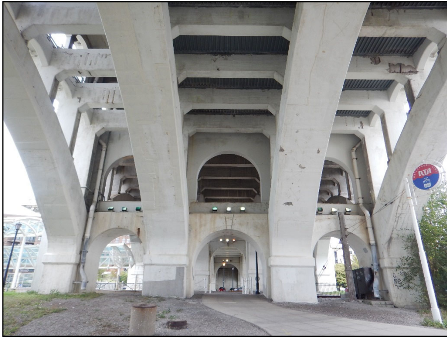
Photo 40 – Pier, typical condition
