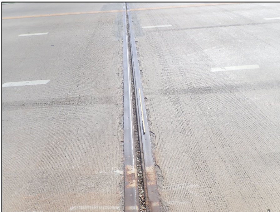
Photo 6 – Typical expansion joint condition
