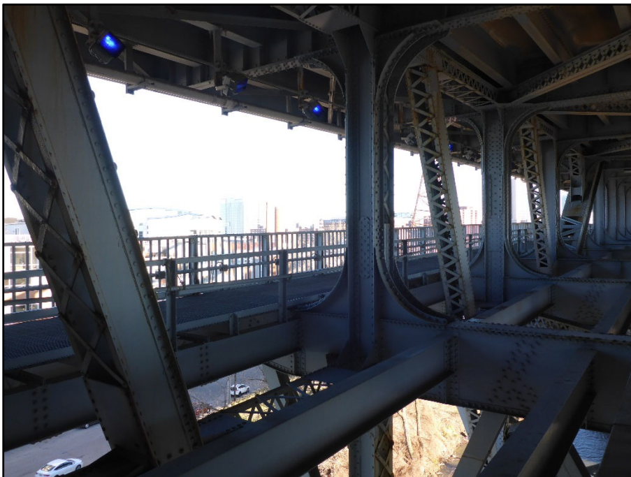
Photo 27 – Typical truss condition
