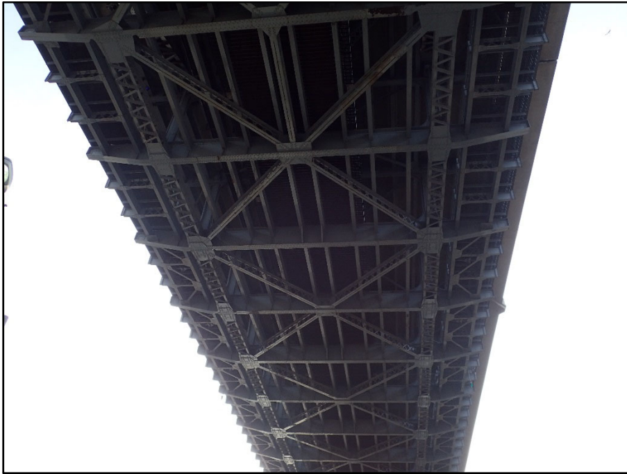
Photo 26 – Typical superstructure condition
