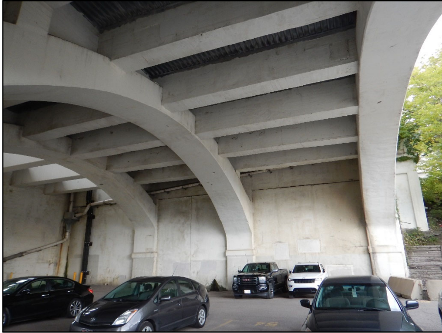
Photo 36 – East Abutment typical condition
