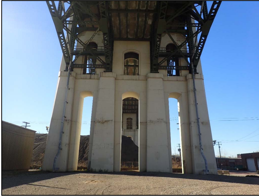
Photo 21 – Pier typical condition
