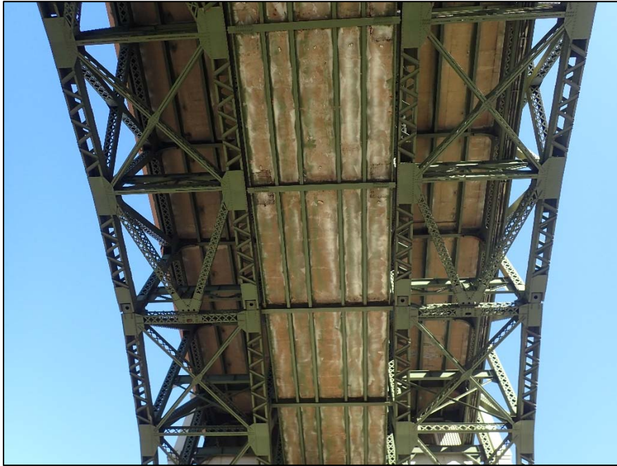
Photo 1 - Typical upper and lower deck soffits
