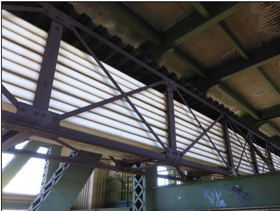
Photo 28 – Typical Telecom conduits
