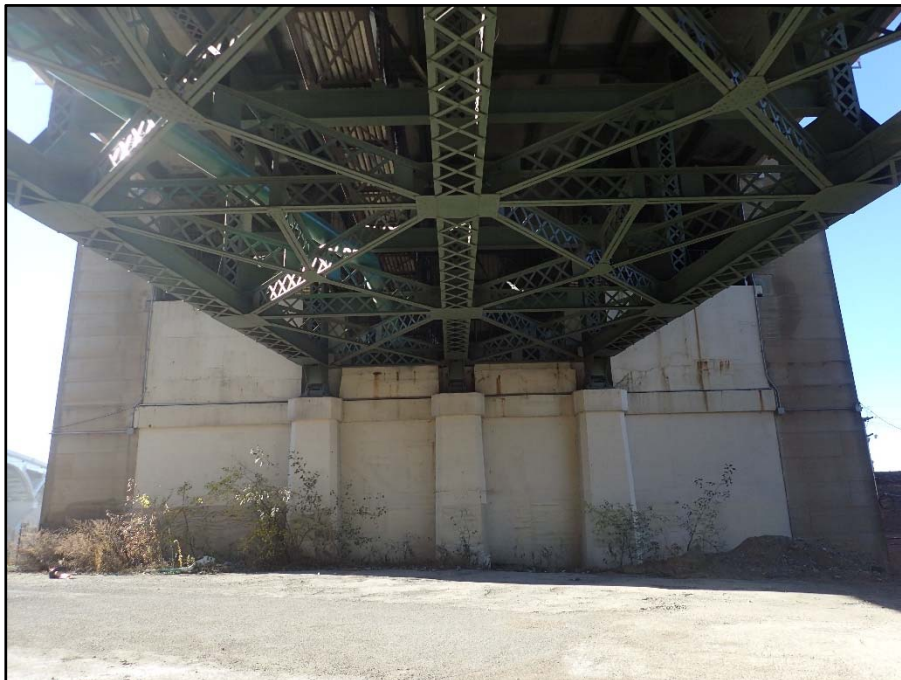
Photo 20 – East Pylon, East face; Typical condition
