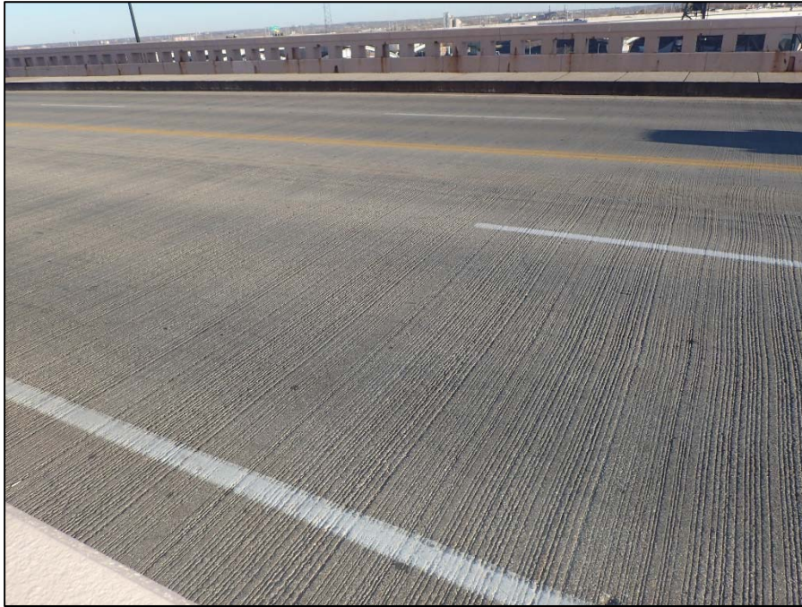
Photo 3 – Typical wearing surface condition
