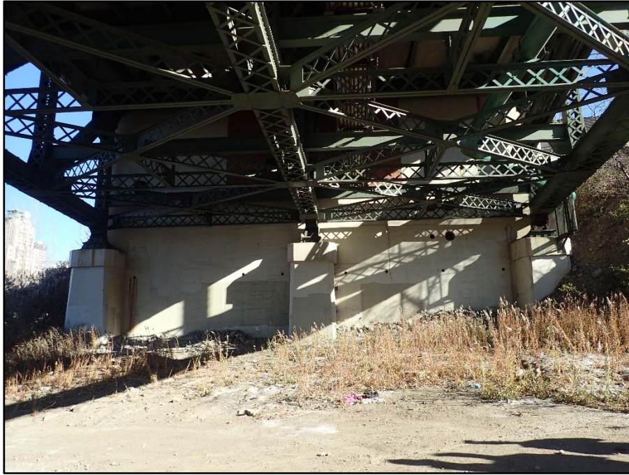
Photo 19 – East Abutment typical condition
