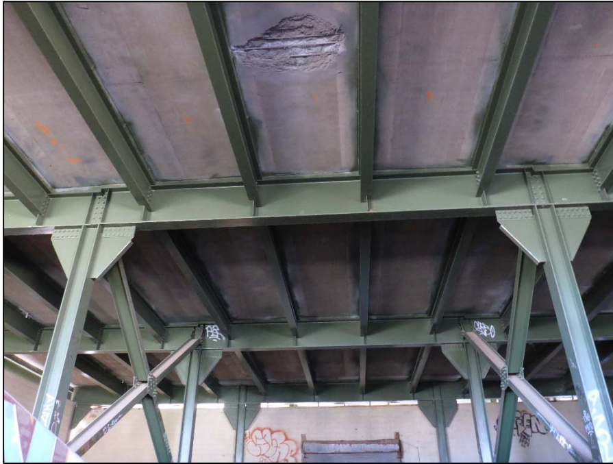
Photo 11 – Typical West approach superstructure
