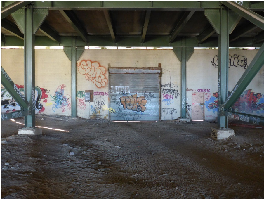
Photo 28 – West Abutment typical condition
