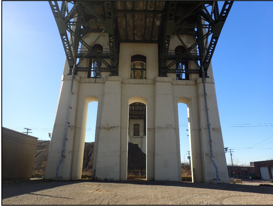
Photo 27 – Pier typical condition
