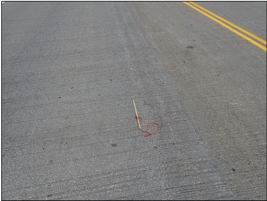
Photo 3 – Typical wearing surface condition
