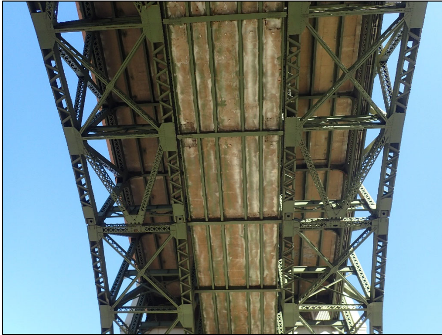
Photo 1 - Typical upper and lower deck soffits
