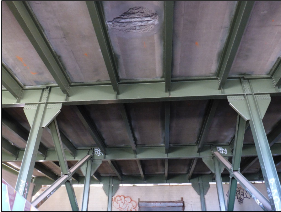
Photo 11 – Typical West approach superstructure
