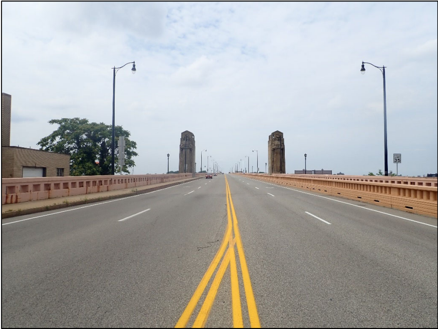
East end view looking West
