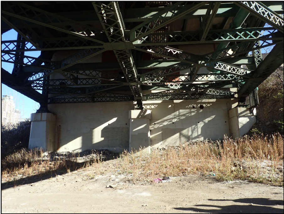
Photo 25 – East Abutment typical condition
