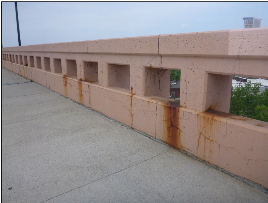
Photo 6 – Typical bridge rail condition
