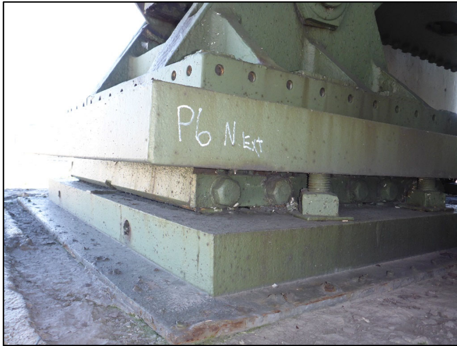
Photo 21 – North Exterior Truss, Pier 6; Typical nested rocker bearing
