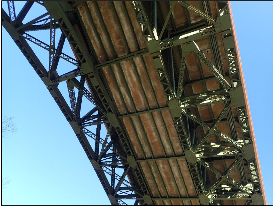
Photo 9 – Typical superstructure condition
