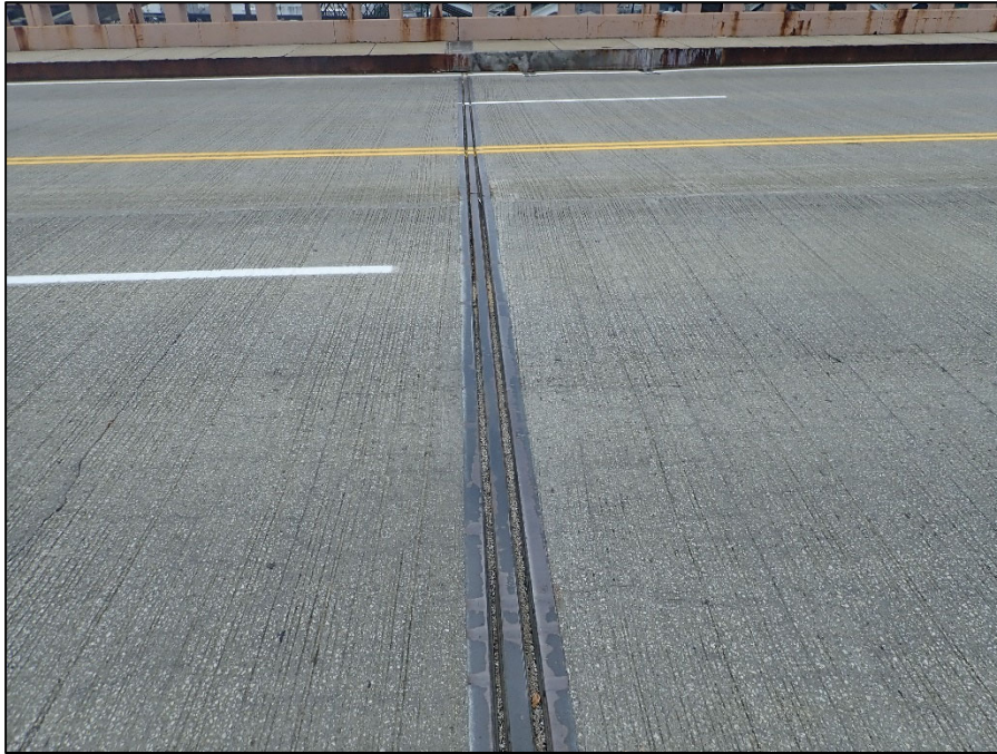
Photo 7 – Typical expansion joint condition
