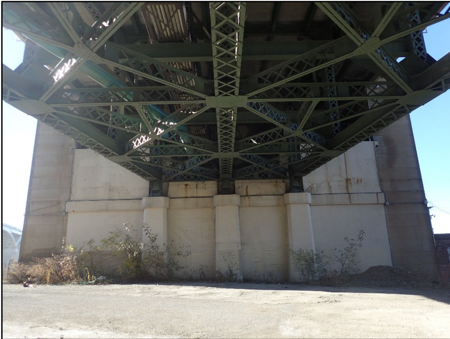
Photo 26 – East Pylon, East face; Typical condition
