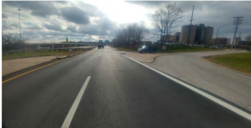
Looking Southbound From North Leg
