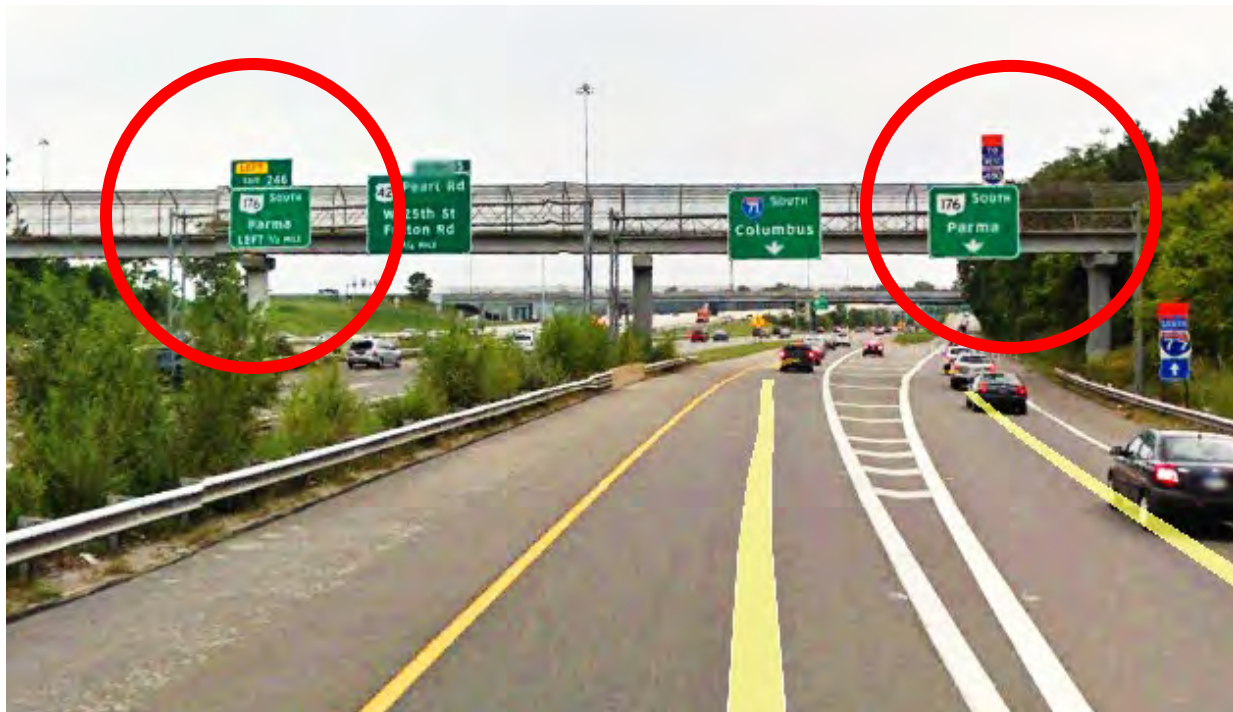
PHOTO 2: C-D ROAD GUIDE SIGNS FOR SB SR176
