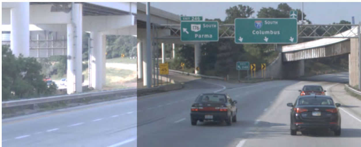
Figure 2- I-71 SB to SR-176 Exit Ramp (SLM 18.04) (July 31, 2012)
