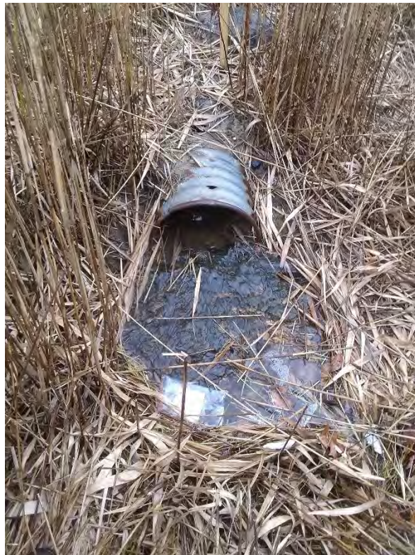
Photo 40. PIP 23 – 11/25/20 – Clear Water, No Odor
