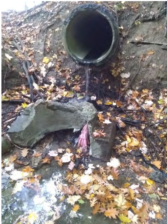
Photo 16. PIP 10 – 10/15/20 – Clear Water, No Odor
