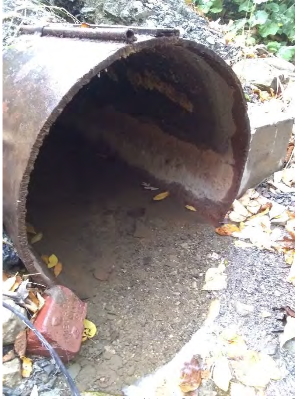
Photo 13. PIP 9 – 10/15/20 – Clear Water, No Odor
