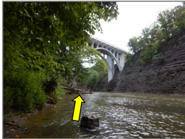
Photo 37 – Looking towards the bridge from upstream (looking north towards Span H). Note the curve in the channel alignment at the bridge and the downed tree.
