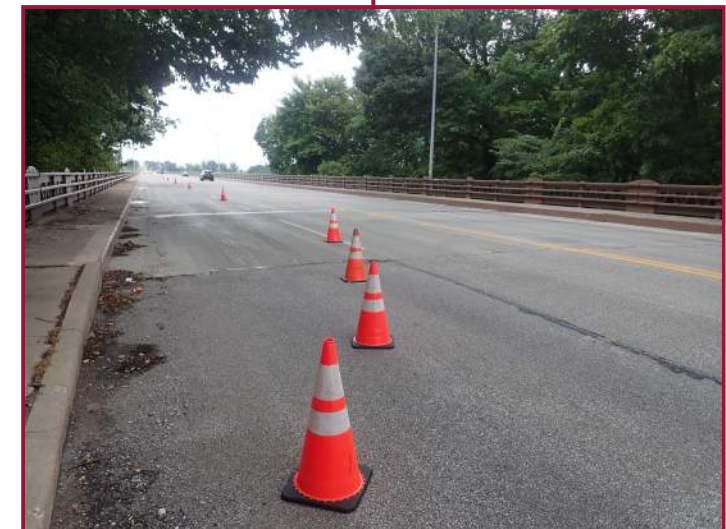
View of the wearing surface from the rear approach (looking east).
