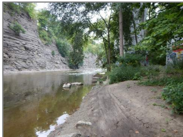
Photo 38 – Looking toward Pier 12 from downstream (looking south). Note the rip rap in the channel near the right column and the proximity of the rear bank.
