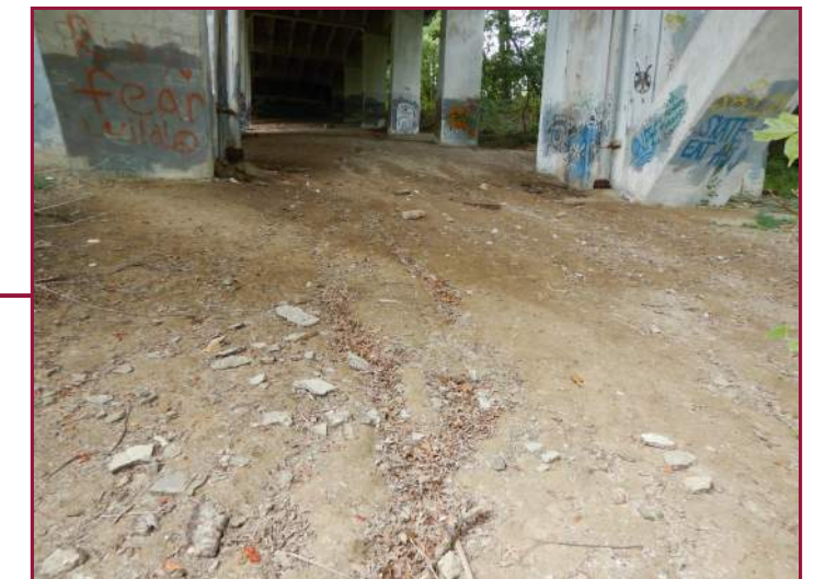
Typical minor erosion channels in the area below the bridge (looking west).
