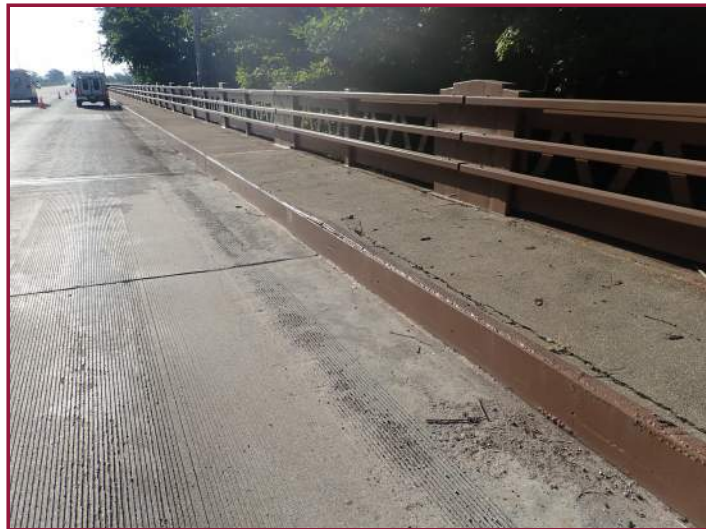
Typical railing and wearing surface (looking southeast from the rear approach).
