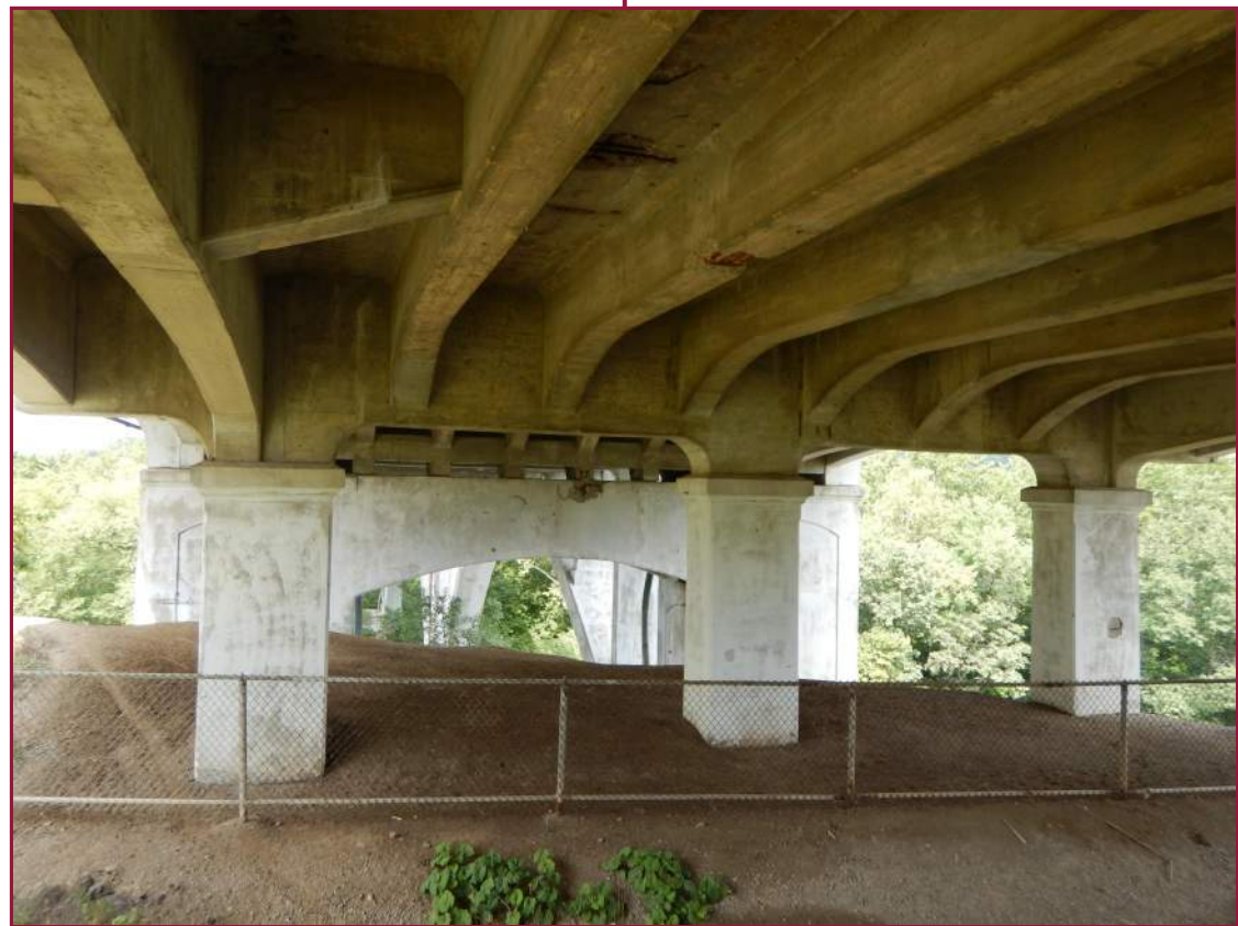
Pier 13 east elevation (looking west).
