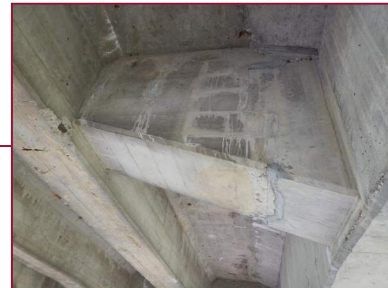
Typical approach span diaphragm (looking west).
