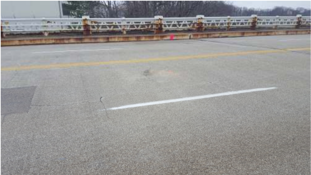
Pavement Photo C-8
