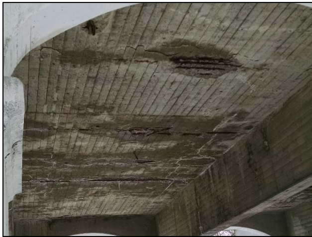
Photo 20 – Interior Bay 2 of Arch A viewed from the south.
