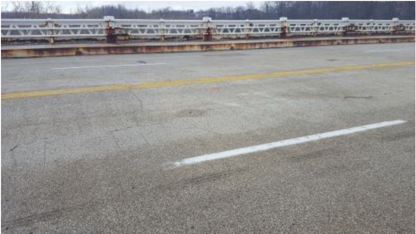
Pavement Photo C-9
