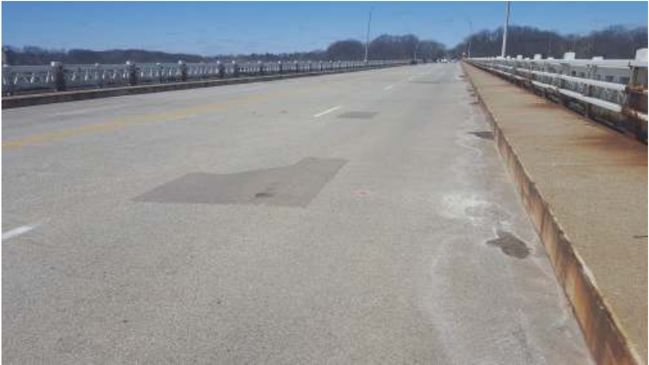
Pavement Photo C-1
