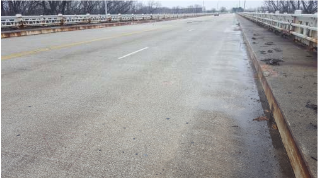
Pavement Photo C-4
