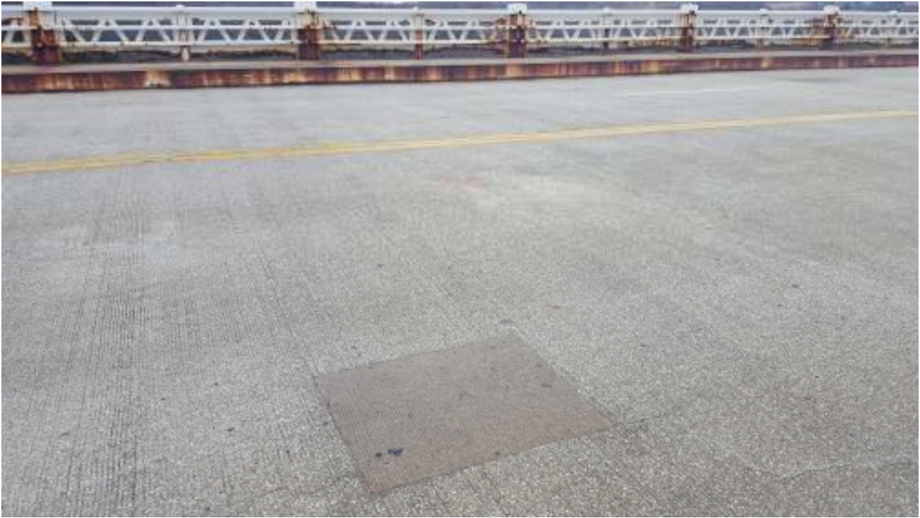
Pavement Photo C-13
