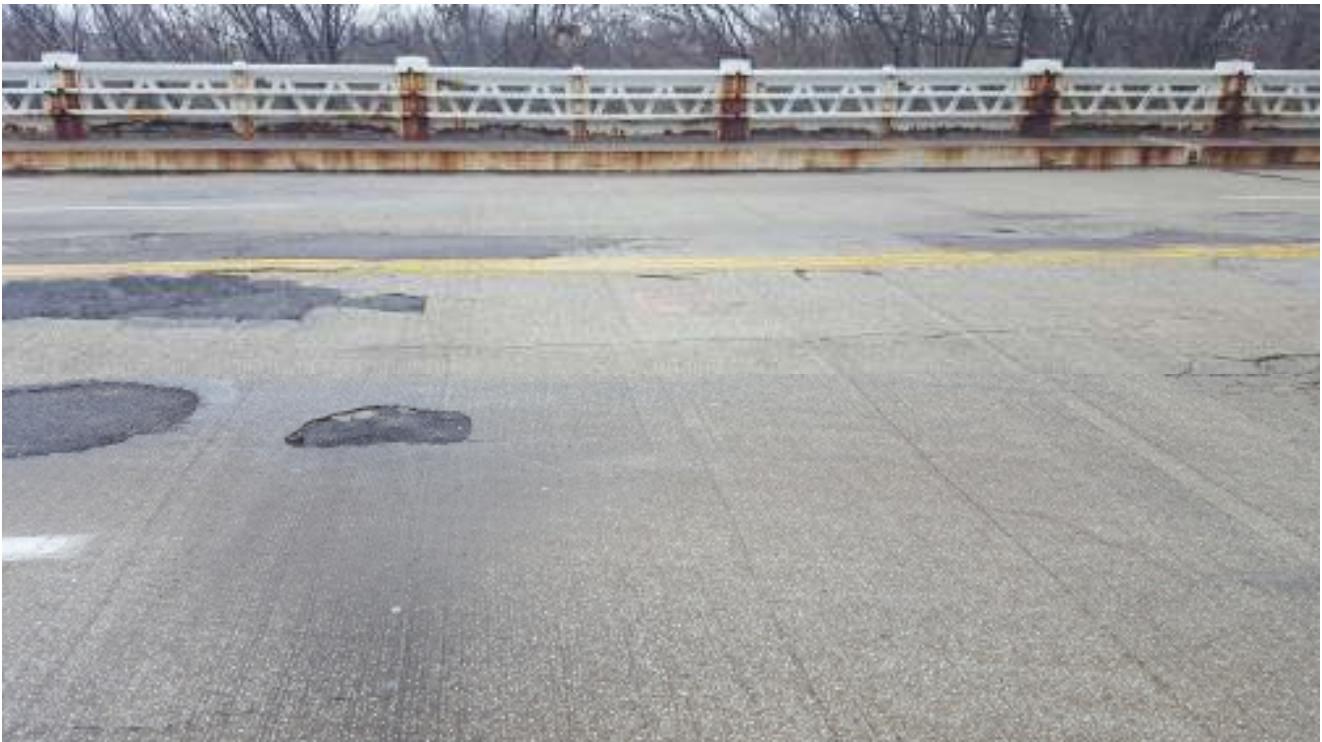
Pavement Photo C-14
