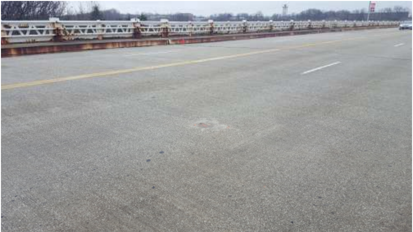
Pavement Photo C-5
