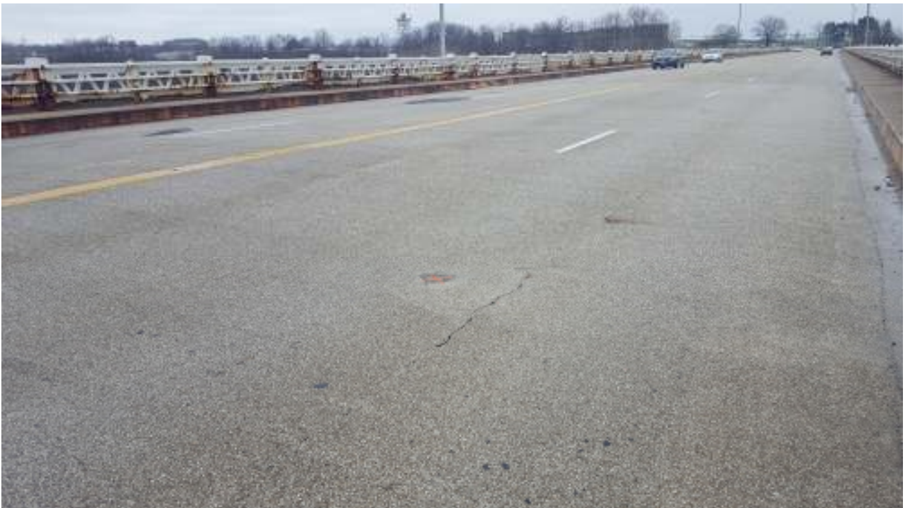
Pavement Photo C-6
