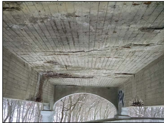
Photo 21 – Interior Bay 4 of Arch A viewed from the south.
