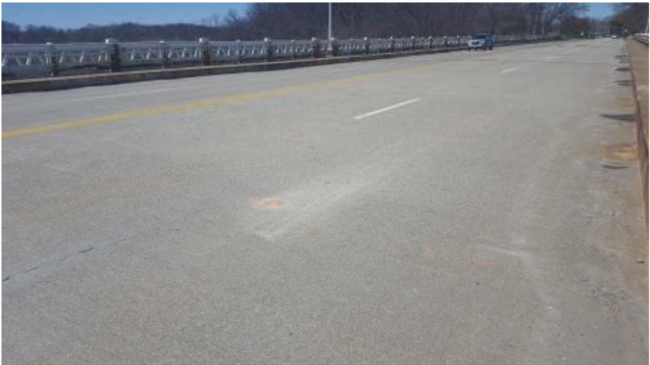
Pavement Photo C-2
