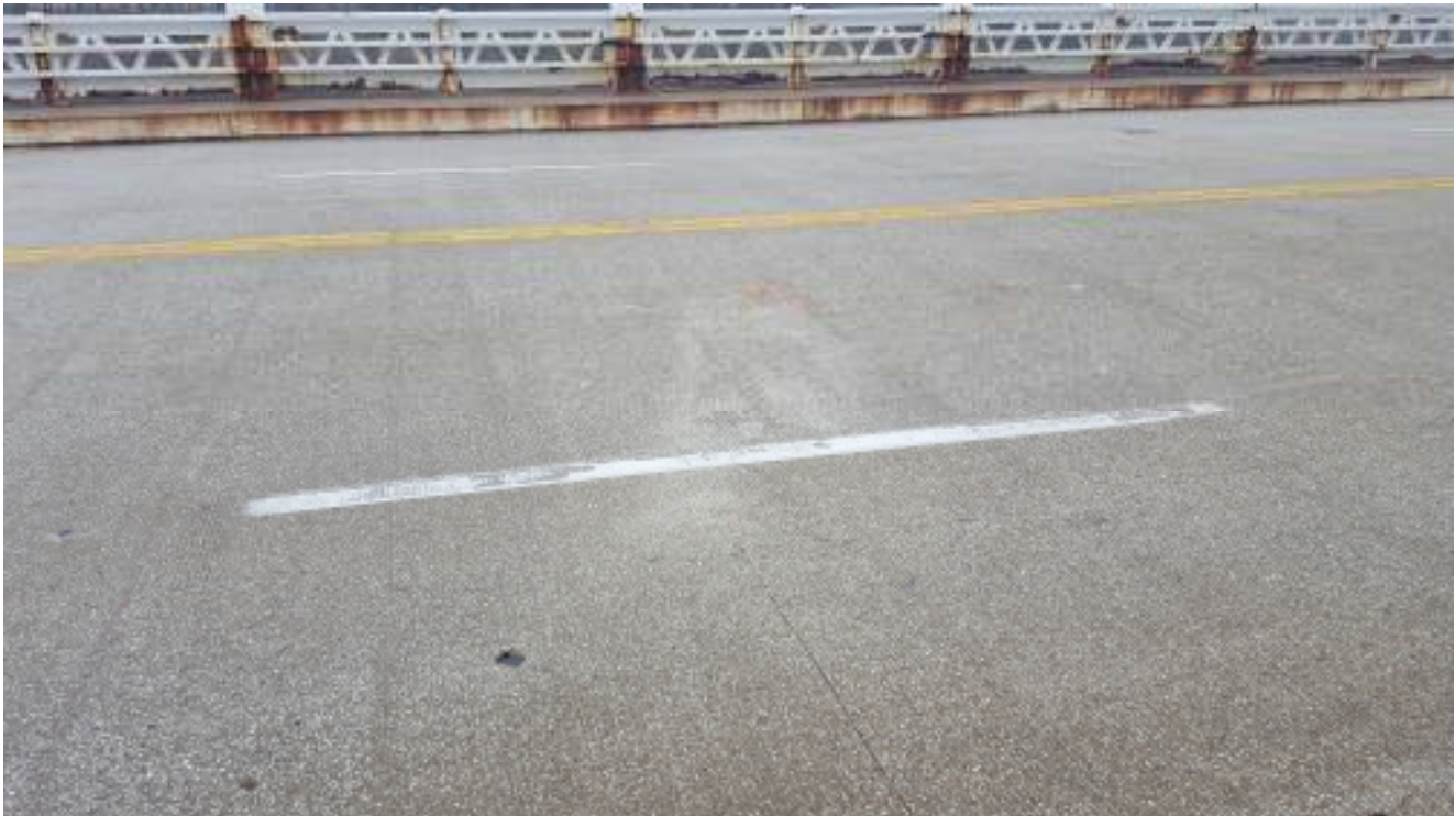
Pavement Photo C-10
