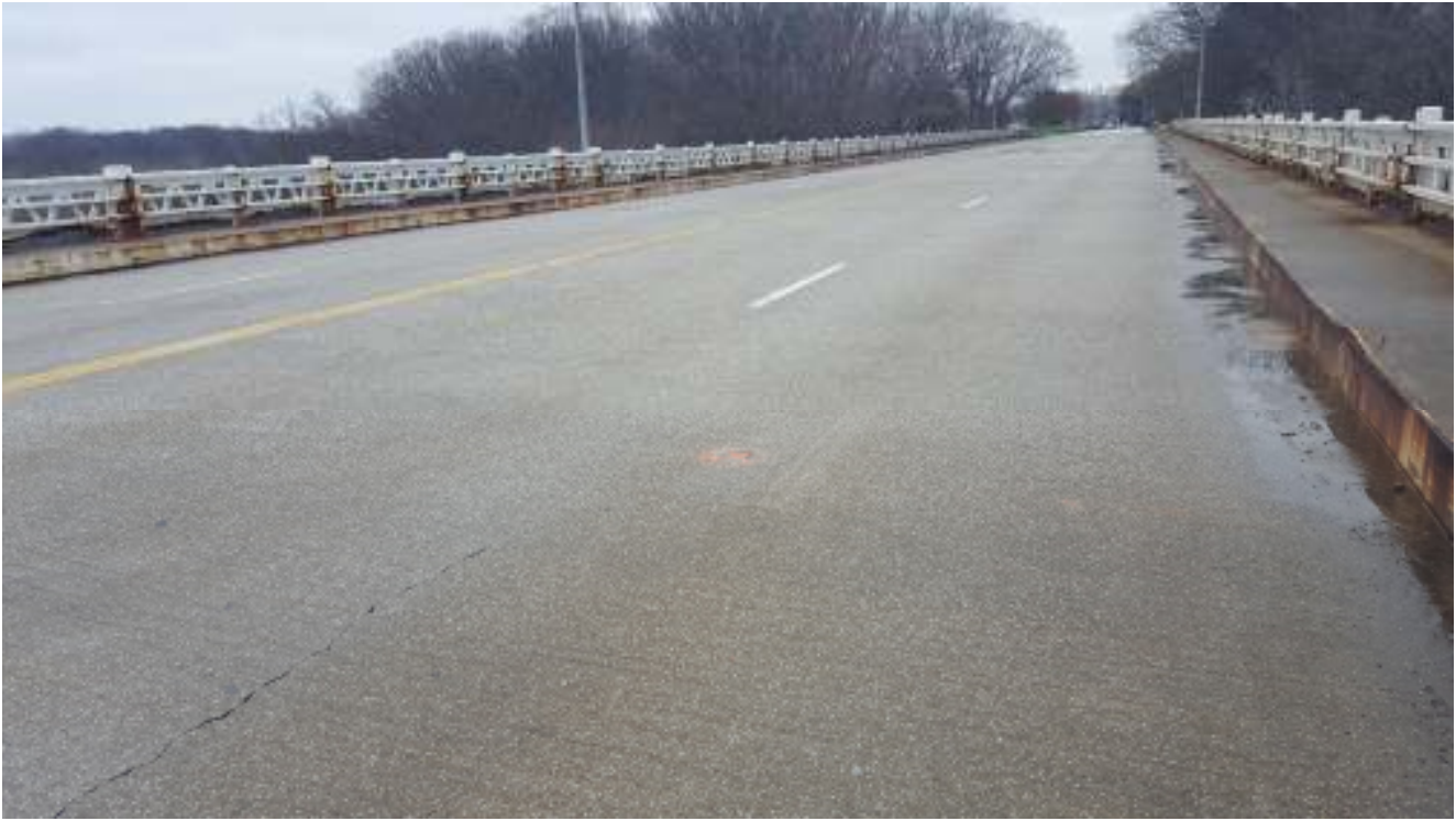
Pavement Photo C-3
