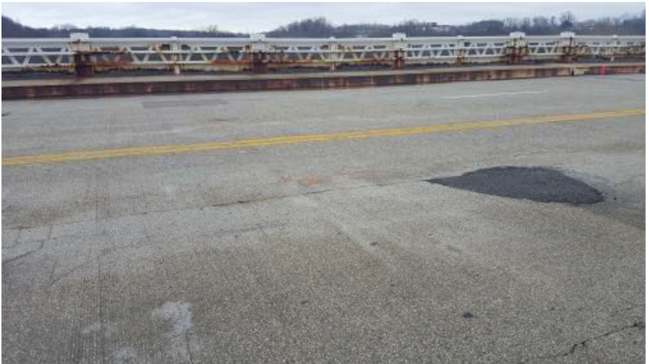
Pavement Photo C-11
