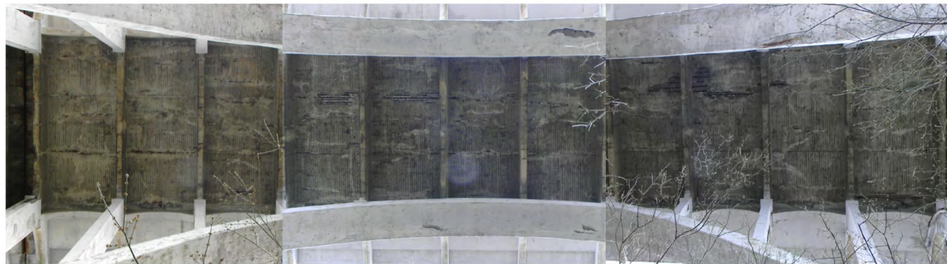
ARCH D - BOTTOM OF DECK PHOTO
