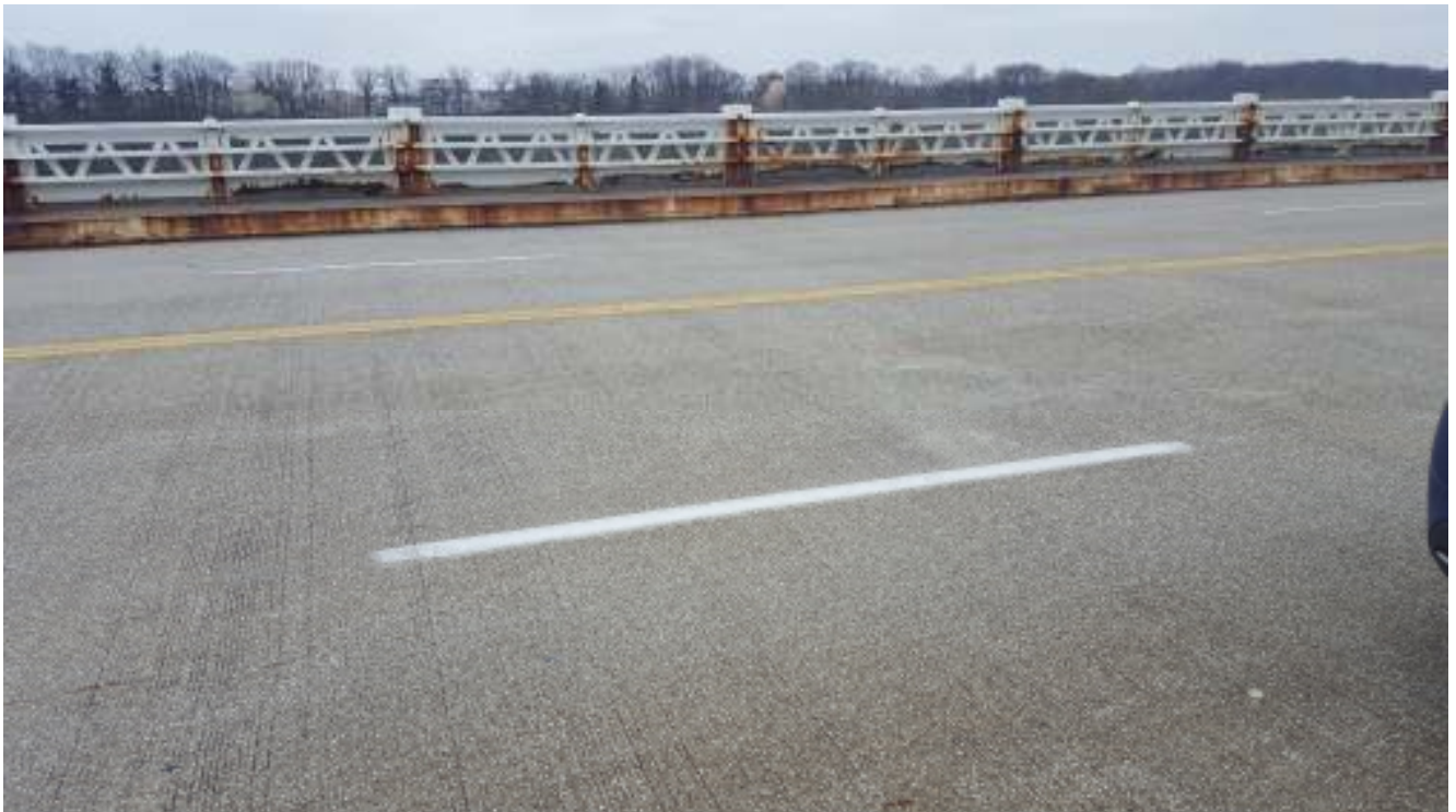
Pavement Photo C-12
