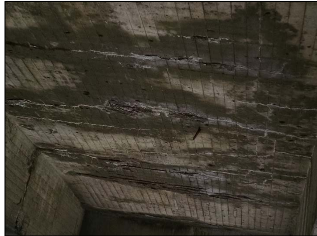
Photo 19 – Interior Bay 1 of Arch A viewed from the south.
