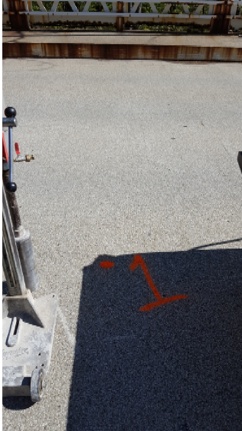
Pavement Photo C-2
