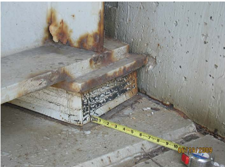
P1: BEARING PAD #1 AT START HAS SHIFTED AS MUCH AS 1.25"
