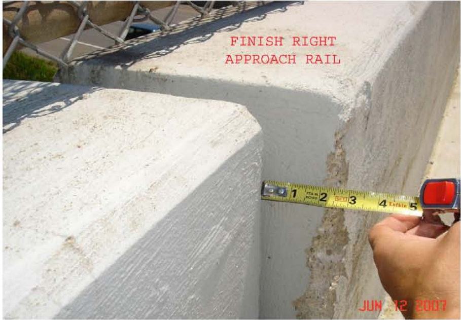
P3: AS MUCH AS 2" ROTATION OF THE BRIDGE DECK.
