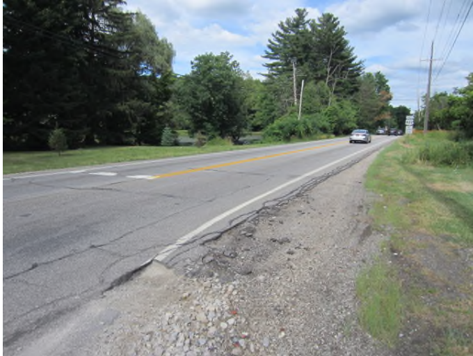
Figure 2. U.S. 422 Looking East
